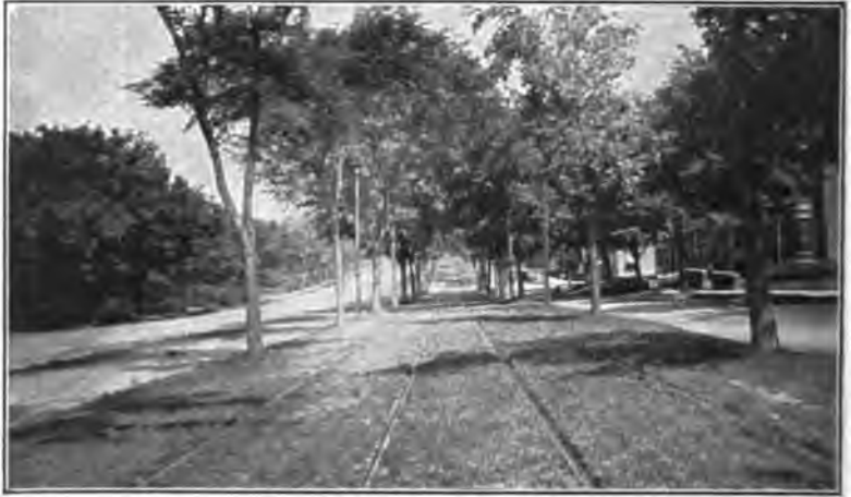
CAR TRACKS ON A CENTRAL RESERVED STRIP—TREE-BORDERED AND SODDED View of a section of Beacon Street, Boston.
