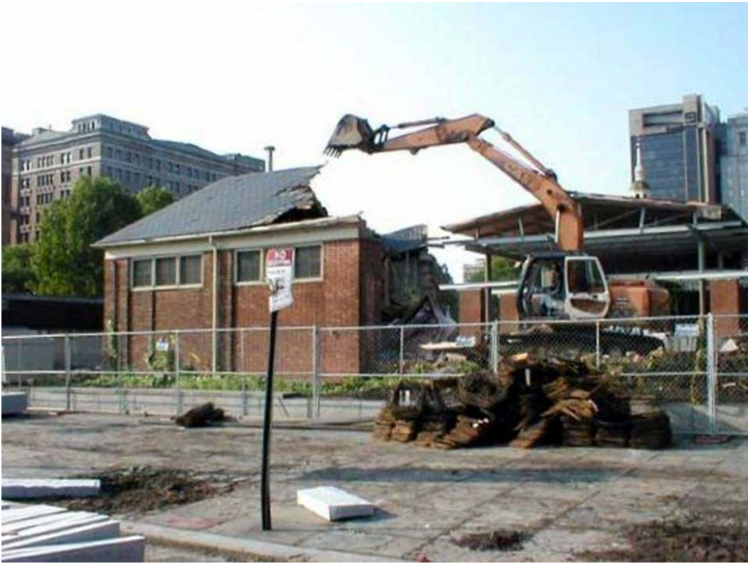
Demolition of the Public Toilet (2003 May 27)
