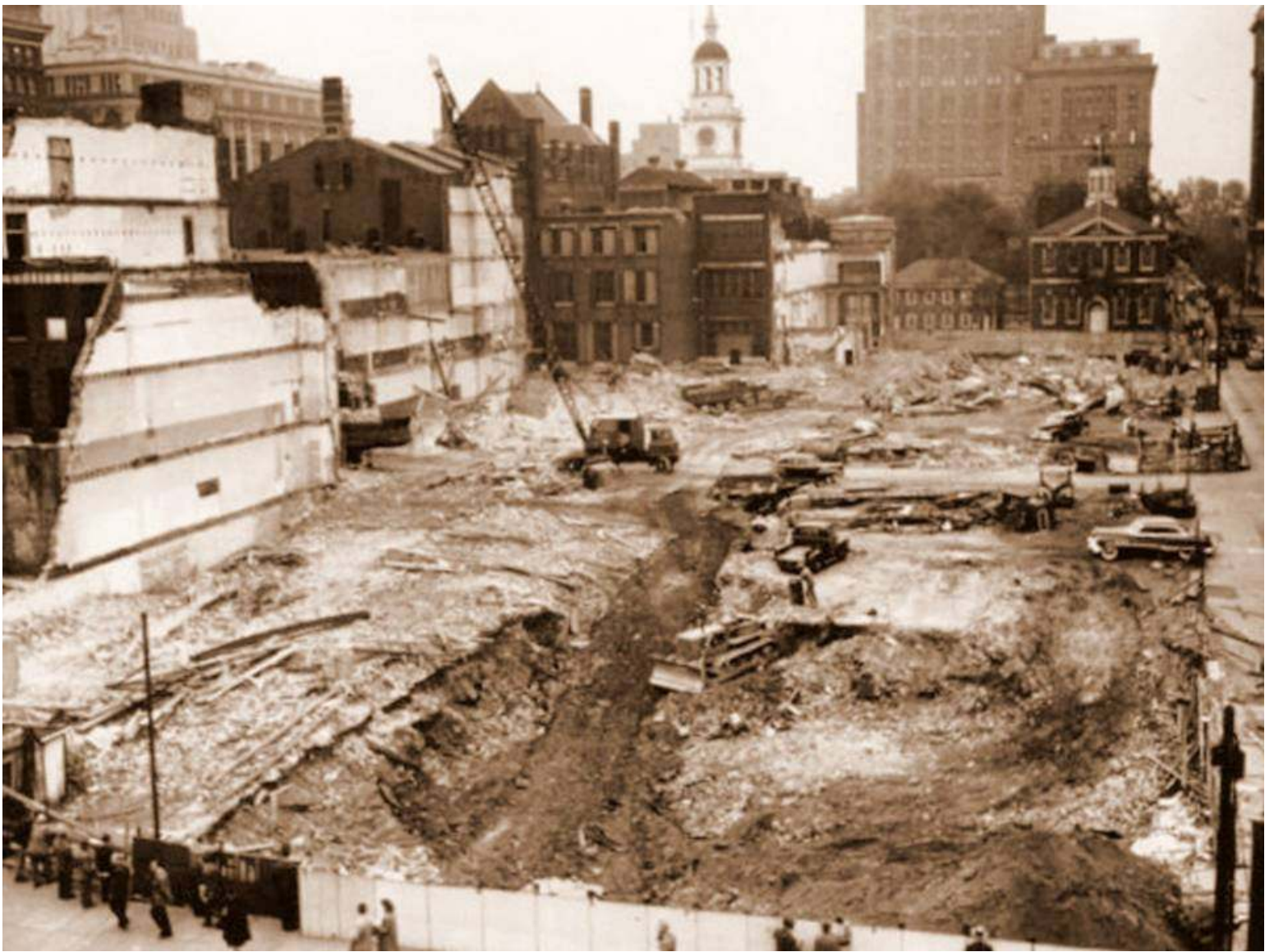
Demolition of 524-36 Market Street (1951 November 1).
