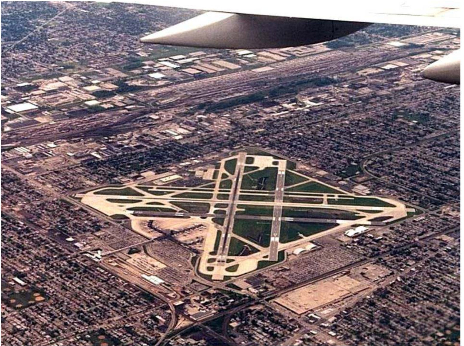
Overview of Midway Airport and the old terminal.
