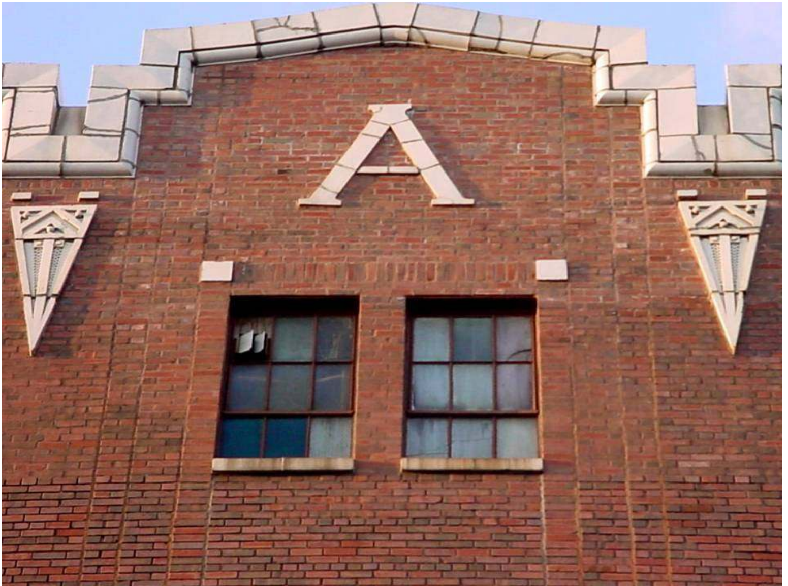
Midland Warehouse. Western Avenue 1500S. Chicago, Illinois. 2005 March 11.
