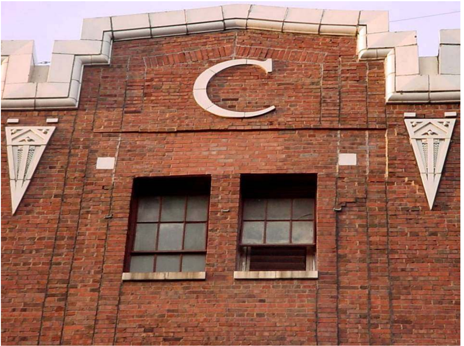
Midland Warehouse. Western Avenue 1500S. Chicago, Illinois. Still working 2005 March 11.
