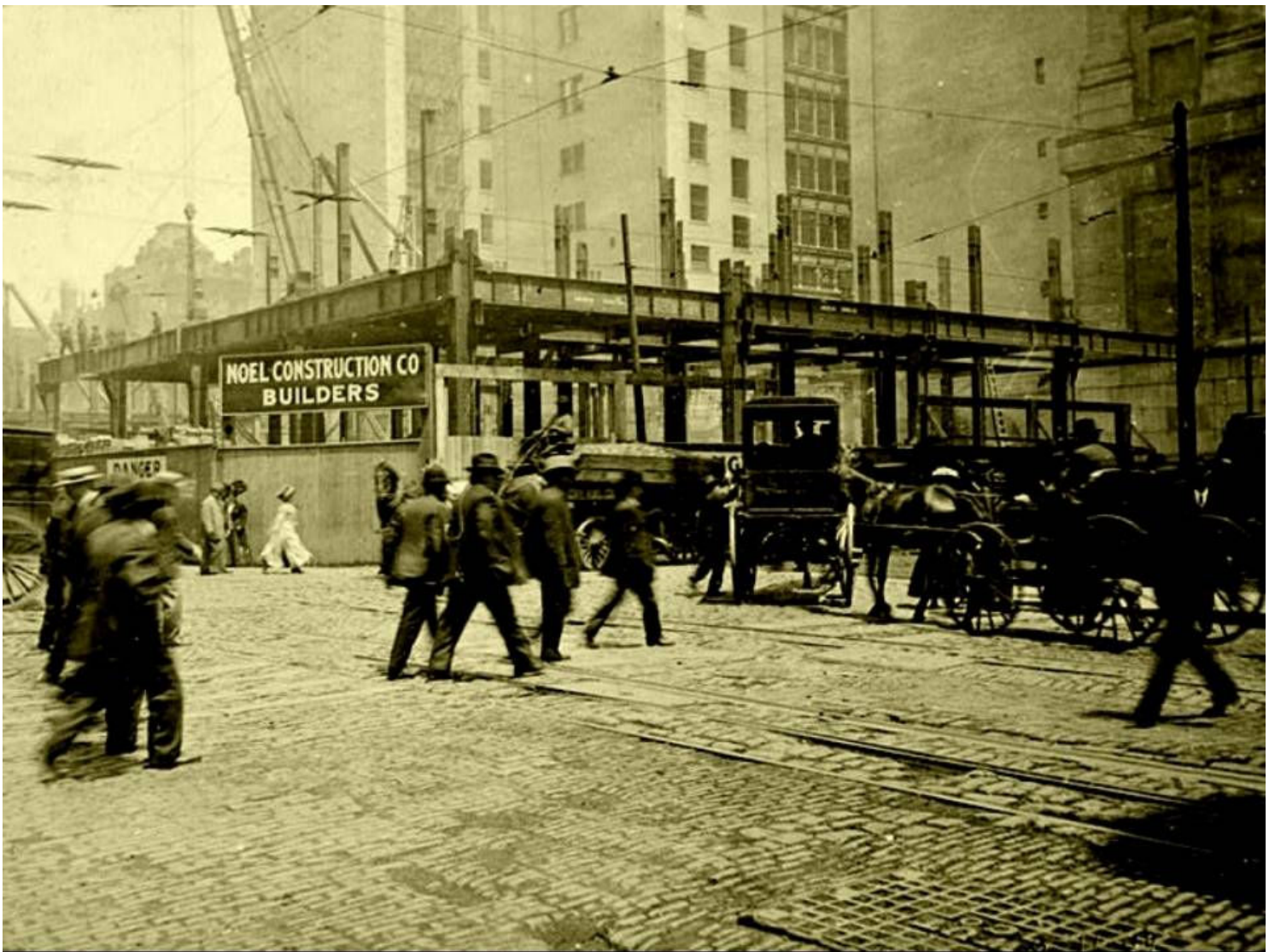
37. First floor skeleton erected, county bldg in background - Chicago City Hall, 121 North LaSalle Street, Chicago, Cook County, IL
