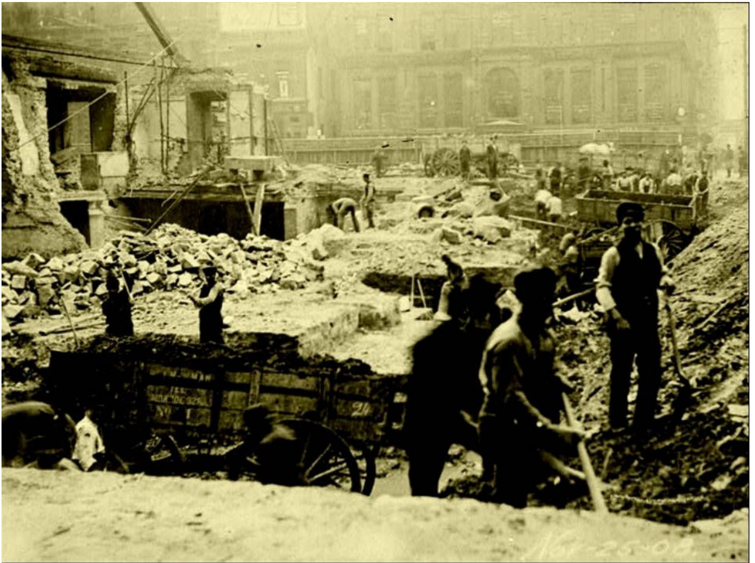
22. Workmen clearing debris - Chicago City Hall, 121 North LaSalle Street, Chicago, Cook County, IL
