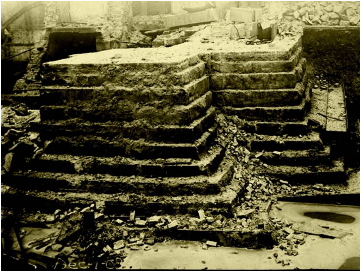
27. Detail of foundations - Chicago City Hall, 121 North LaSalle Street, Chicago, Cook County, IL
