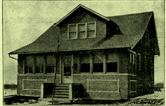
ONE OF THE NEW HOMES JUST COMPLETED.
