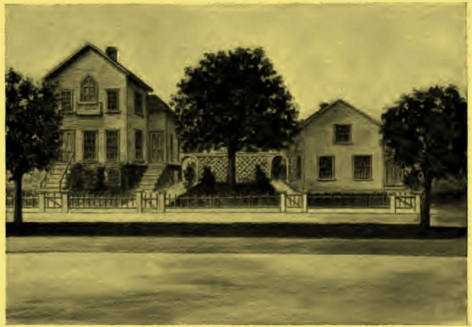
RESIDENCE OF FERNANDO JONES (at the left)
