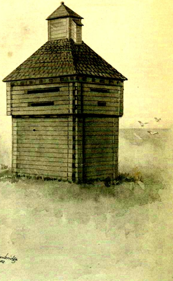
THE FORT DEARBORN BLOCK HOUSE, DEMOLISHED IN 1856.
