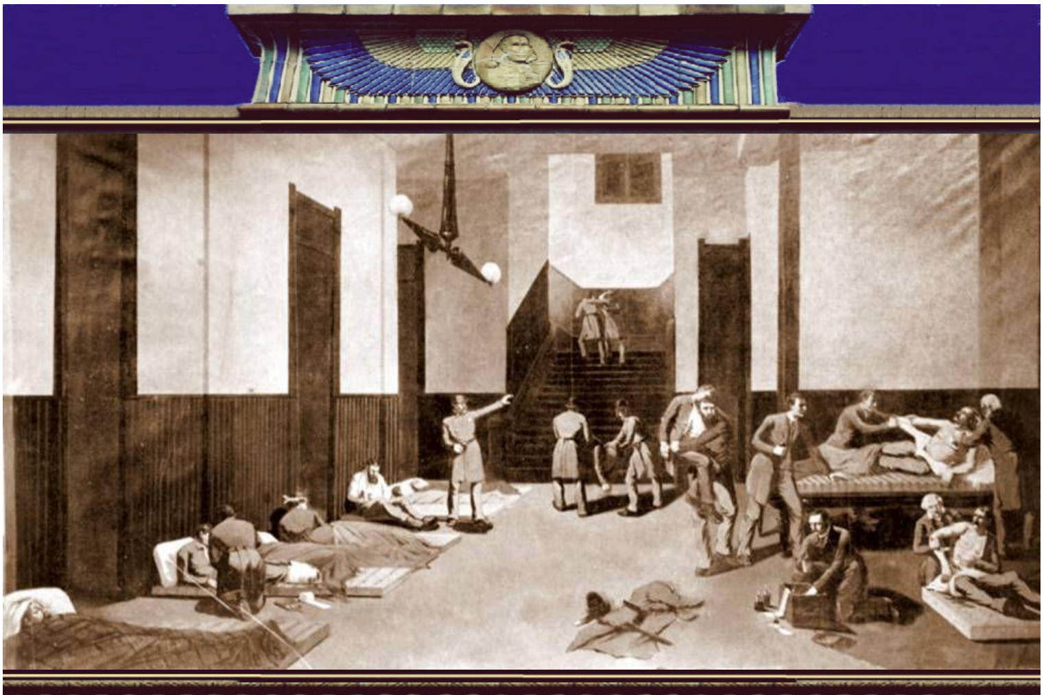
Desplaines Street Police Station after riot at Haymarket Square, Chicago (1886 May 4)
