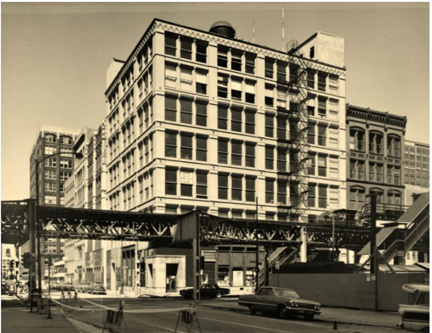
Jenney, William Le Baron (architect). Leiter II Building, State Street (403 South, at East Congress)Streets, Chicago, Cook County, IL
