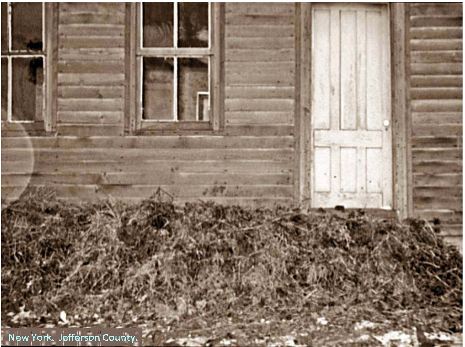
Manure and straw placed around foundation of house for warmth. Jefferson County (NY). Rothstein, Arthur (1915-1985) (photographer) (1937 December)
