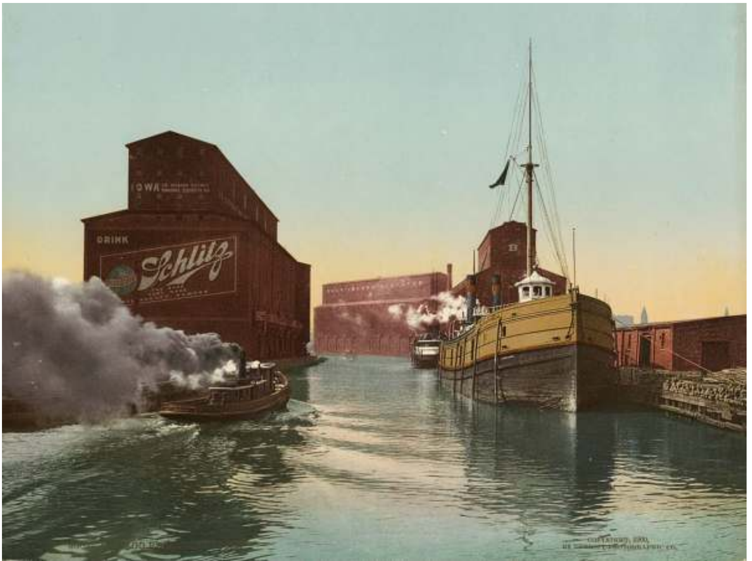
Chicago River elevators. Chicago, Illinois. Detroit (MI): Detroit Publishing Company (copyright 1900).
