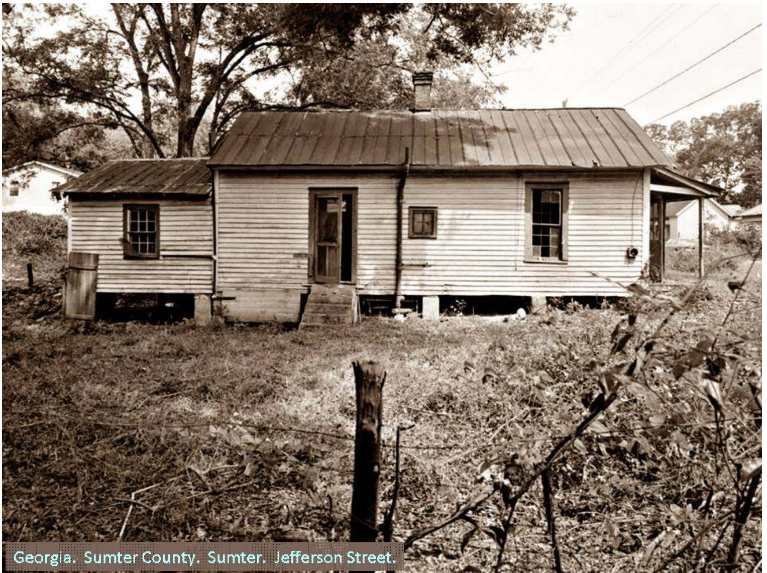
Shotgun house. 304 East Jefferson Street, Sumter, Sumter County (GA). Photo 2 of 8, west side view. HABS GA-2285 (creator/ photographer) (after 1933).
