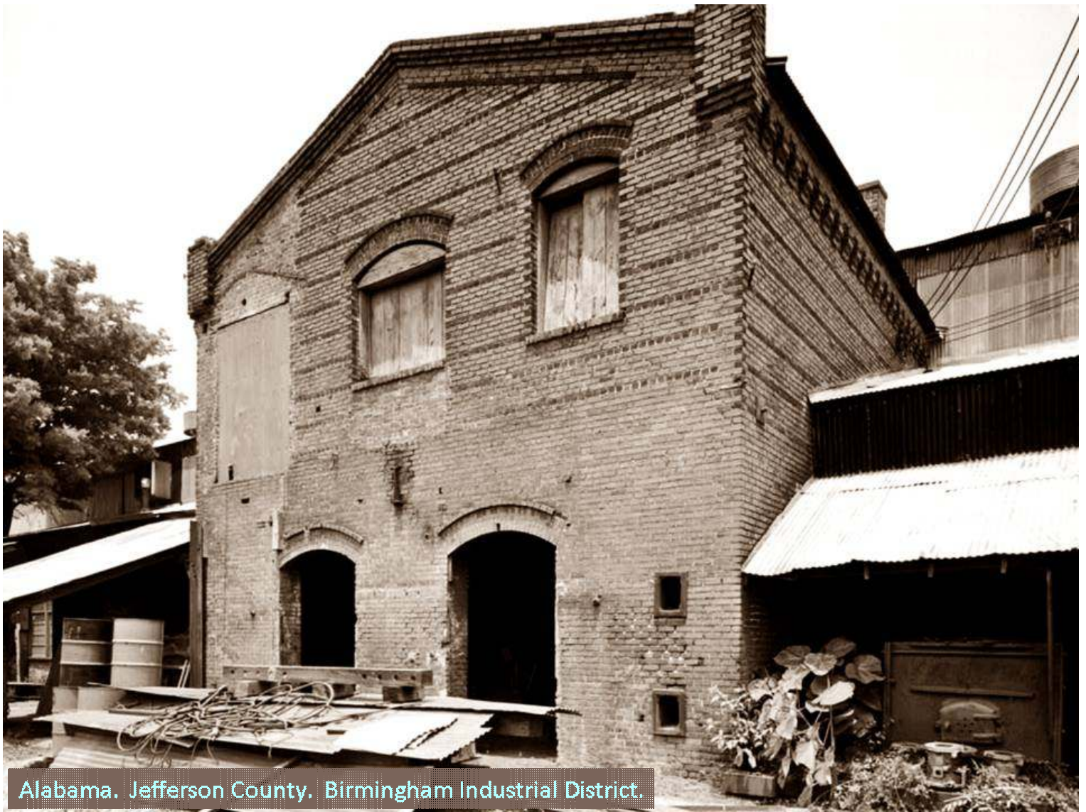
Diesing, David H. (creator) (1992). Erection shop, exterior, west. Hardie-Tynes Manufacturing Company. 800 Twenty-eighth Street North. Birmingham Industrial District. Thomas, Jefferson County, Alabama.
