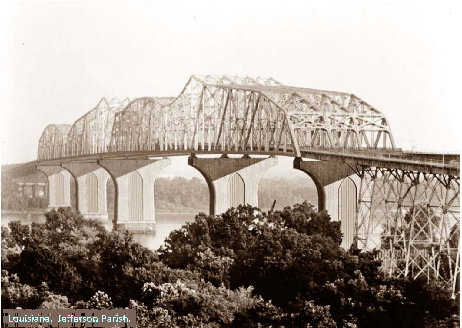
The proposed Huey P. Long Bridge widening, looking from the west bank toward the east bank of the Mississippi River. Photo 213 of 213. HAER LA-17/ Marcus Lamkin (creator/ photographer) (2005)
