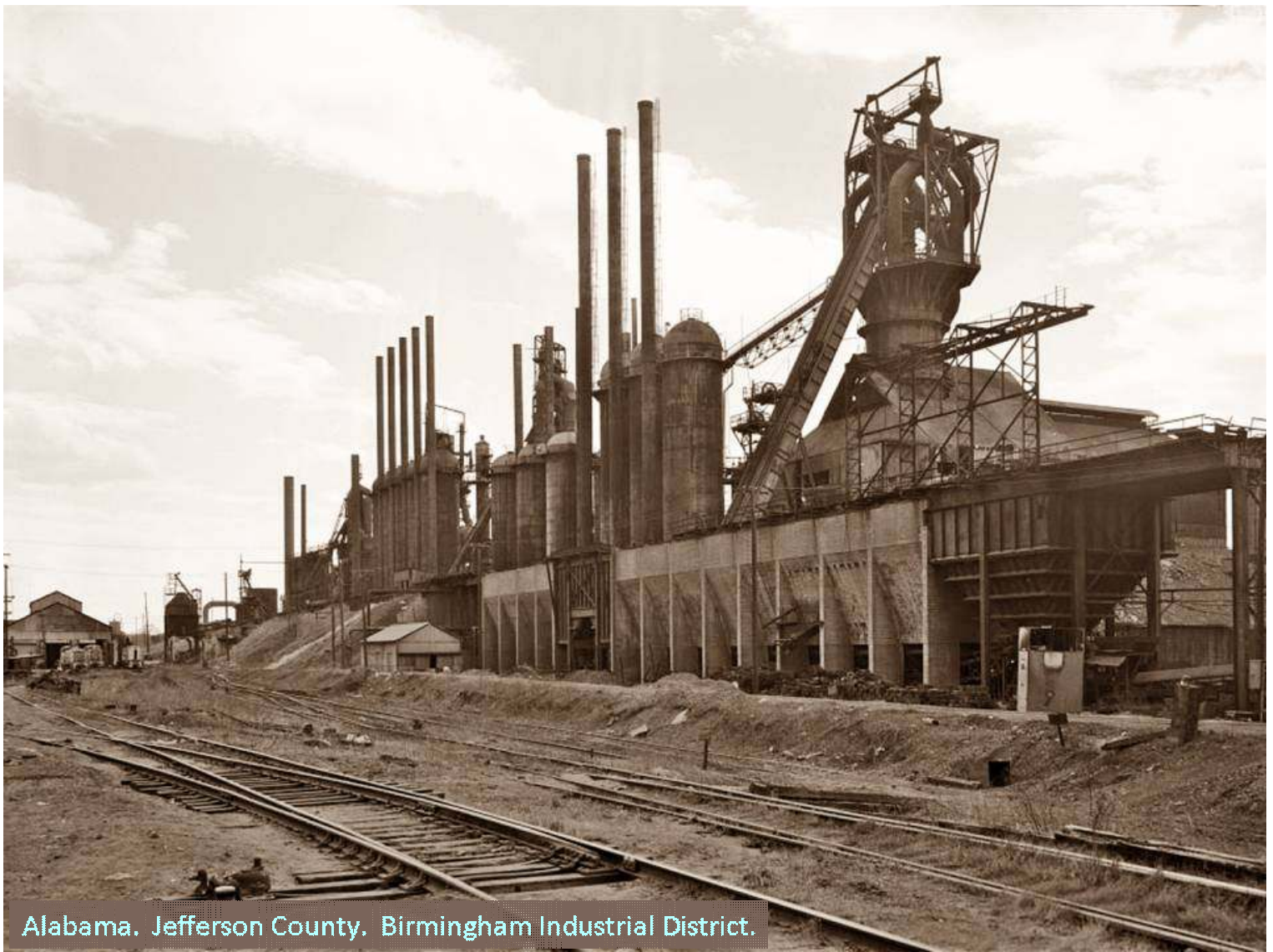
Boucher, Jack E. (photographer) (1974). View from northwest. Woodward Coal & Iron Company Furnace (initial construction 1882). Birmingham Industrial District, Opossum Creek vicinity. Woodward, Jefferson County, Alabama. Photo 4 of 15. HAER AL-4 (after 1968).
