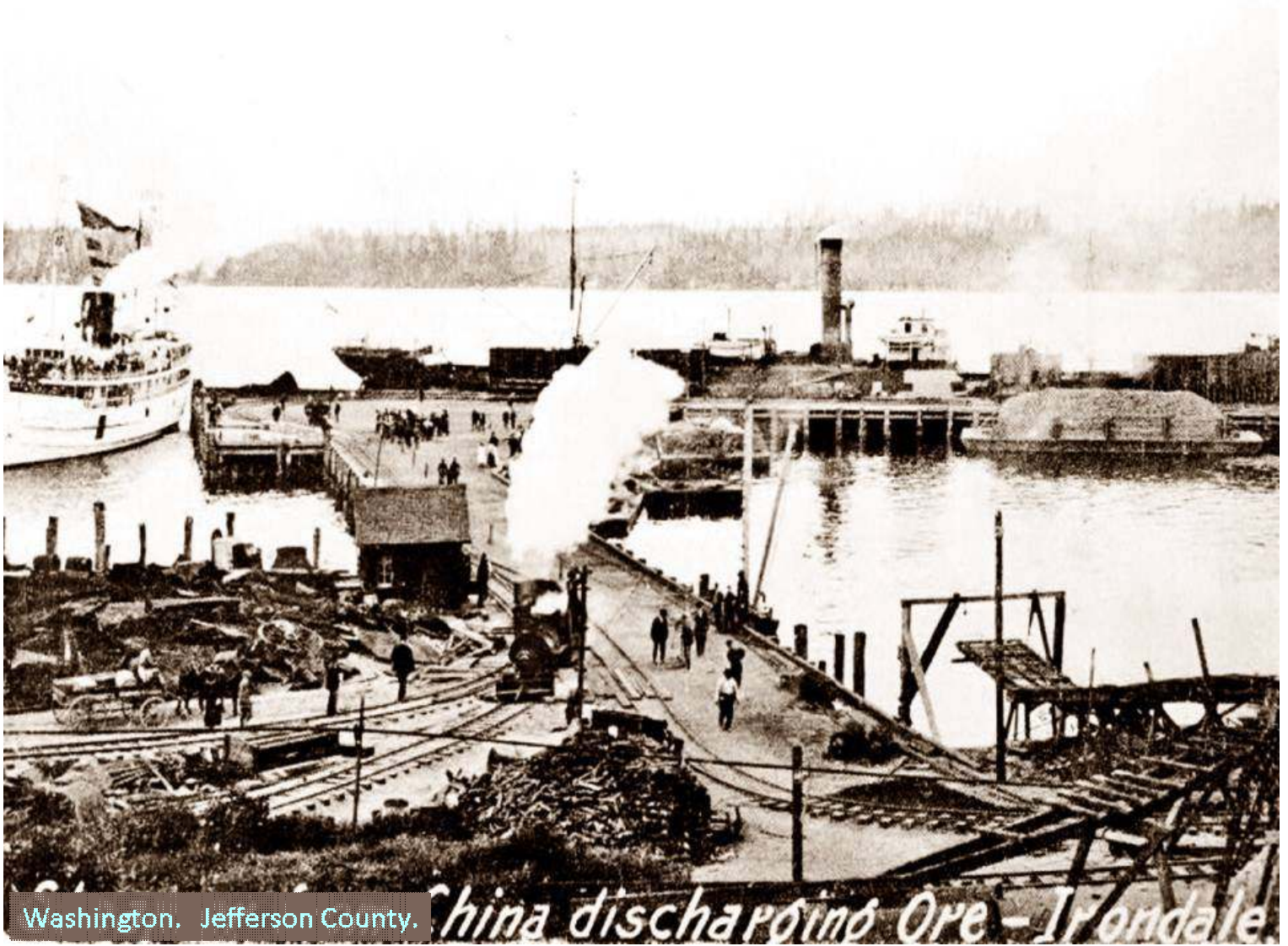
Irondale Iron & Steel Plant. Port Townsend, Jefferson County (WA). Photo 40 of 42, steamer from China unloading ore(1910). HAER WA-7 (creator/photographer) (after 1968).
