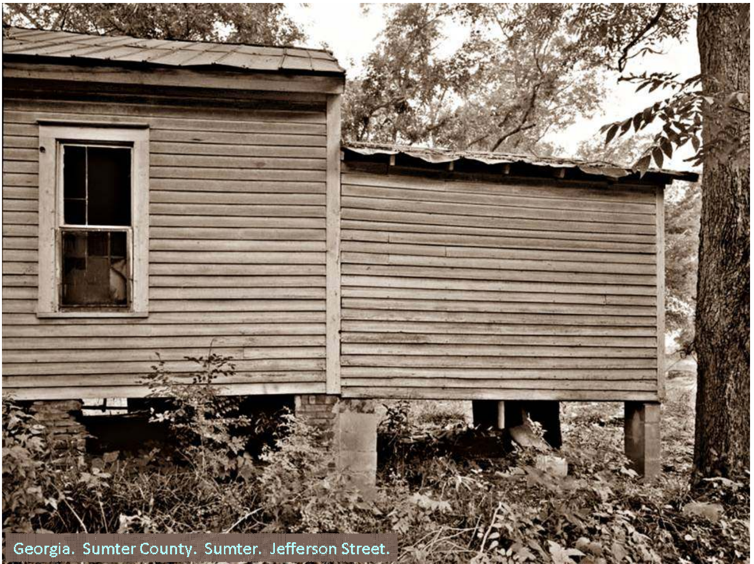
Shotgun house. 304 East Jefferson Street, Sumter, Sumter County (GA). Photo 5 of 8, east and rear side view. HABS GA-2285 (creator/photographer) (after 1933).
