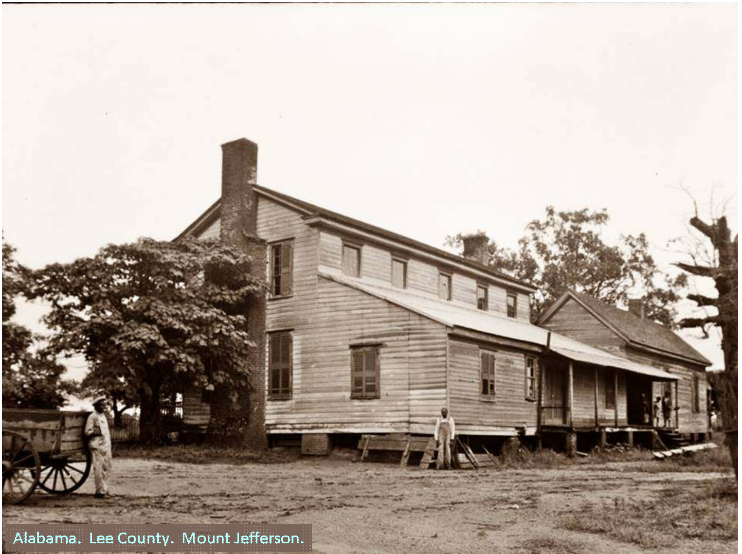
Manning, W.N. (photographer) (1935 September 10). View of rear (west and north sides). Tucker-Fincher House. U.S. Route 431. Mount Jefferson, Lee County, Alabama. Photo 2 of 10. HABS AL-878 (after 1933).
