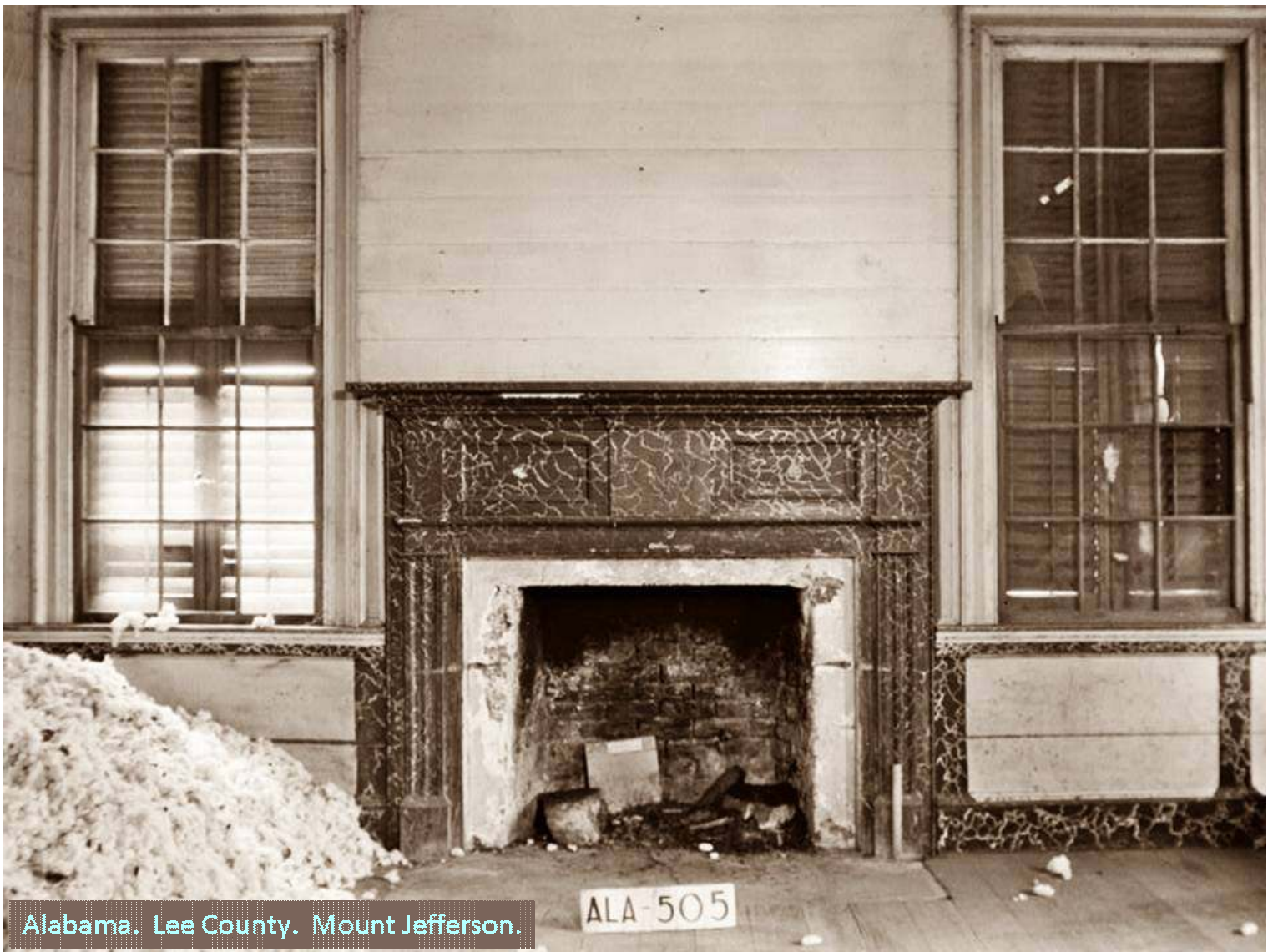
Manning, W.N. (photographer) (1935 September 10). Mantel in parlor (northeast room). Tucker-Fincher House. U.S. Route 431. Mount Jefferson, Lee County, Alabama. Photo 7 of 10. HABS AL-878 (after 1933).
