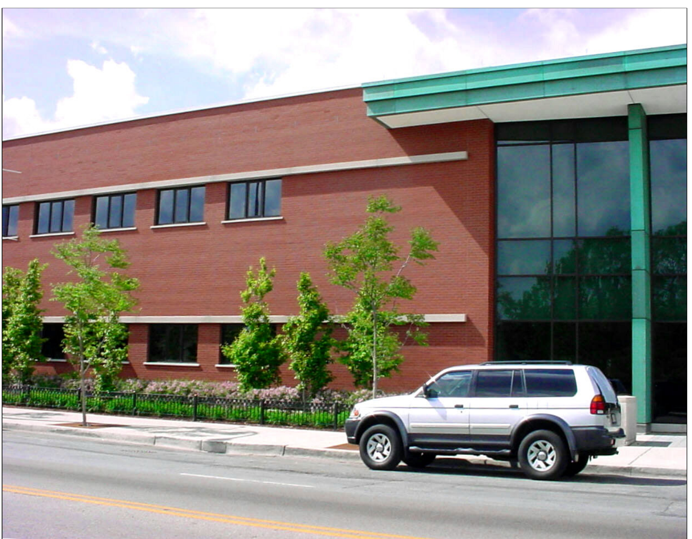
A section of new police station. 63rd Street, Chicago, Illinois.
