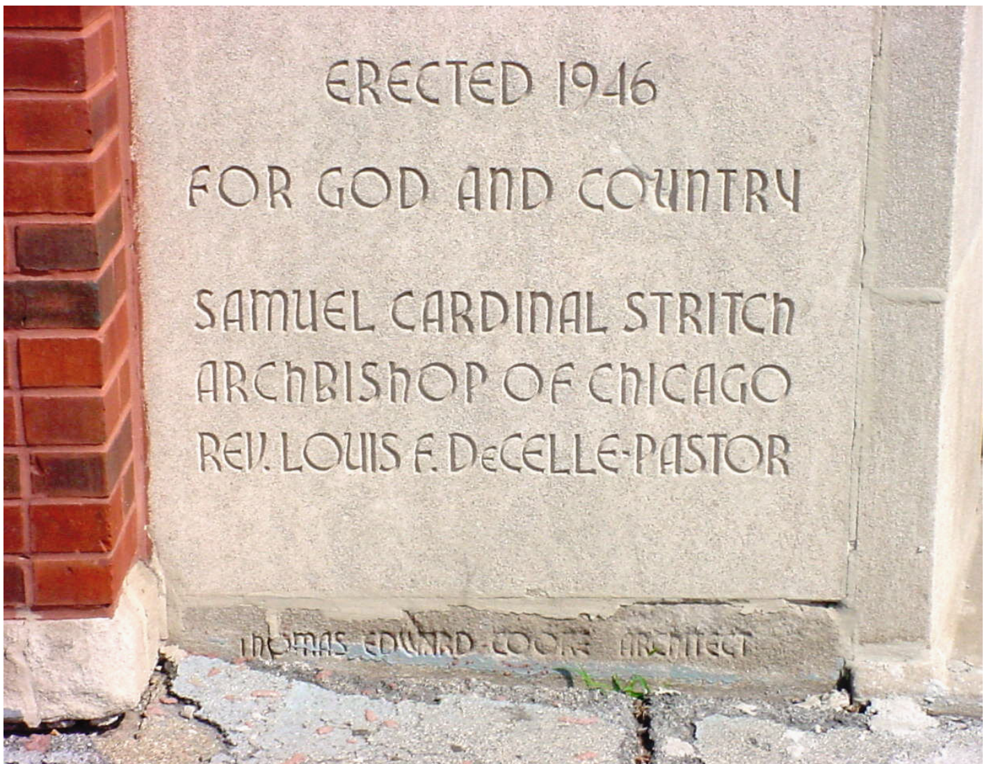
McKinley Park Elementary School, a CPS facility housed in a failed parochial school. Pershing Road (3900S) 2744W, Chicago, Illinois.
