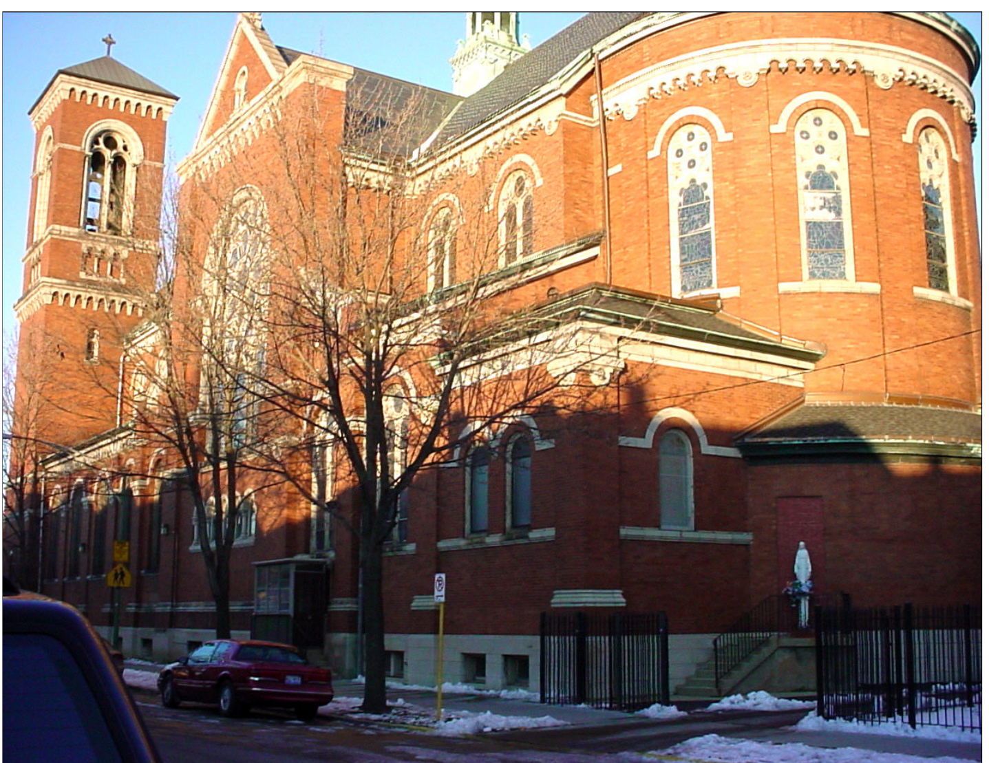
Hermitage Avenue 4831S, Chicago, Illinois.
