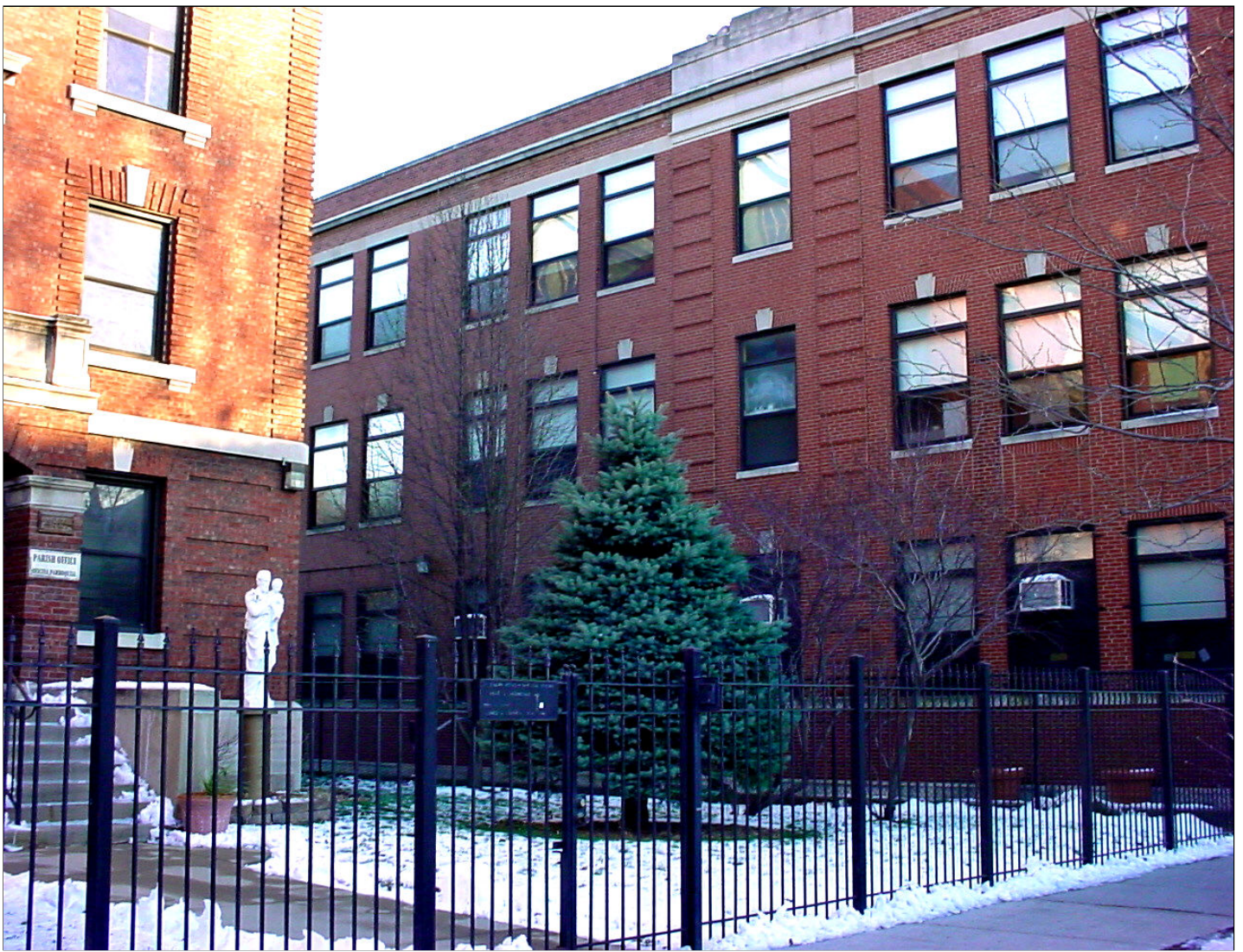
Hermitage Avenue 4831S, Chicago, Illinois.
