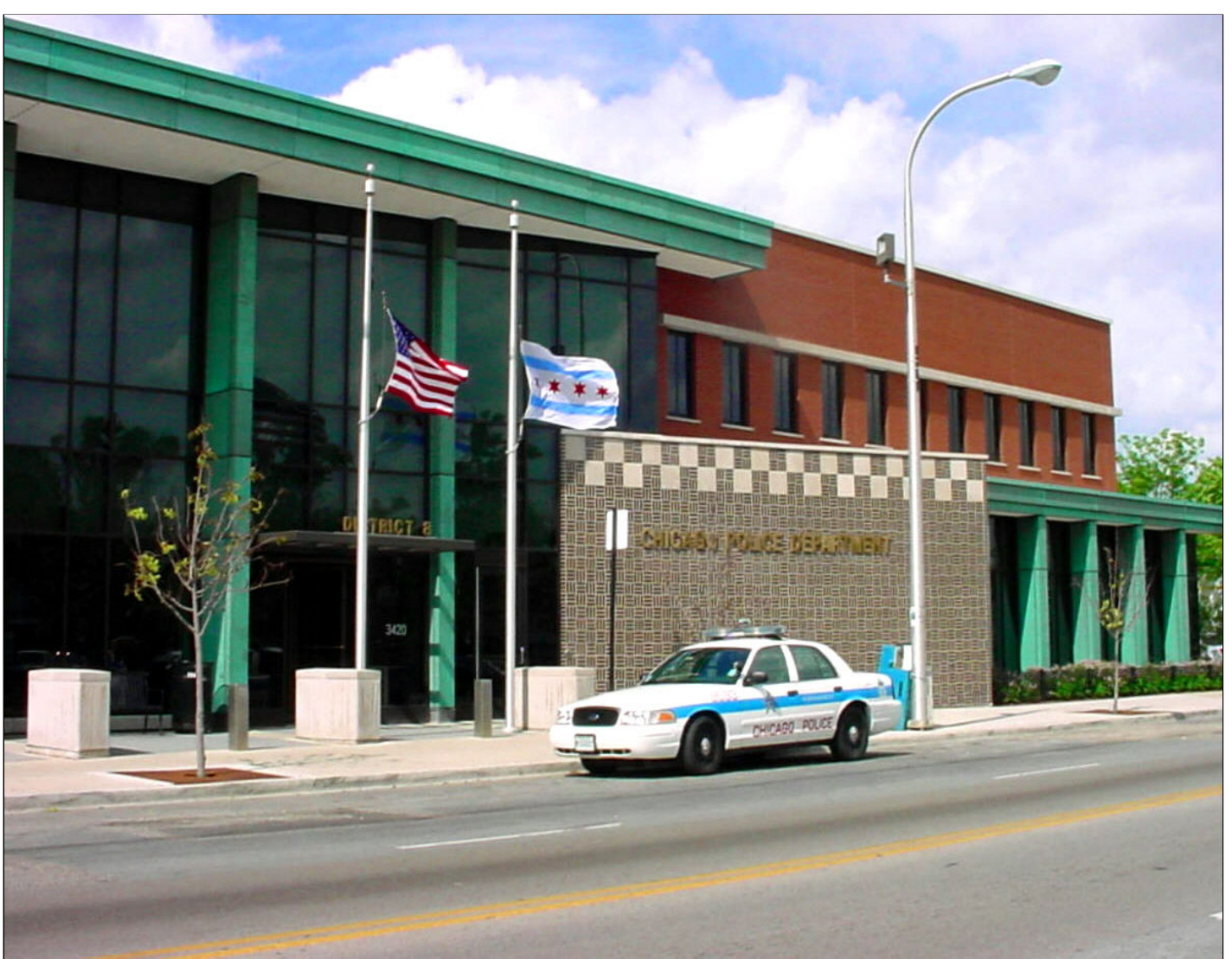
Another section of new police station. 63rd Street, Chicago, Illinois.
