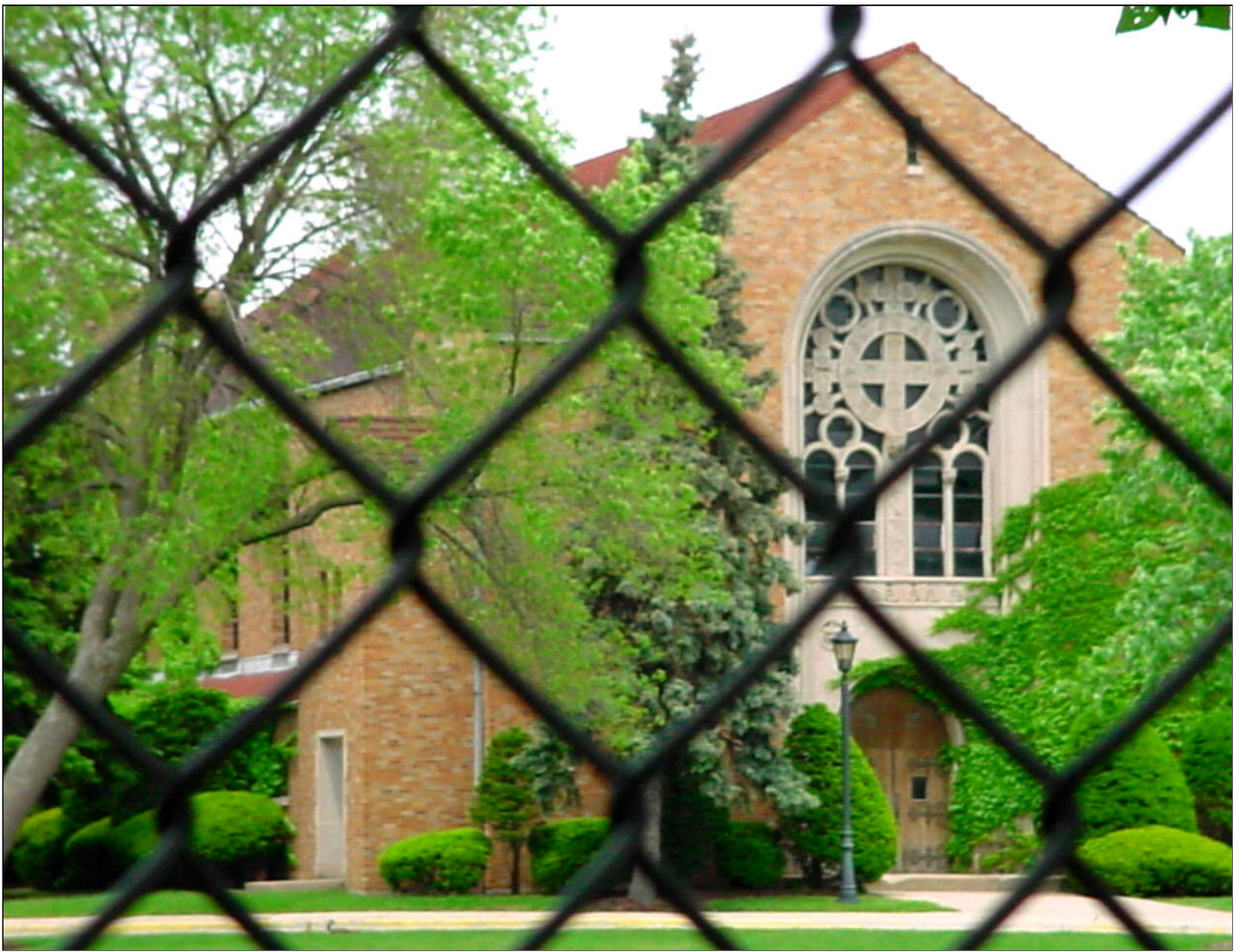
Gwendolyn Brooks Academy, a Chicago Public Schools tax-financed facility. Roseland neighborhood, 111th Street 250E, Chicago, Illinois.
