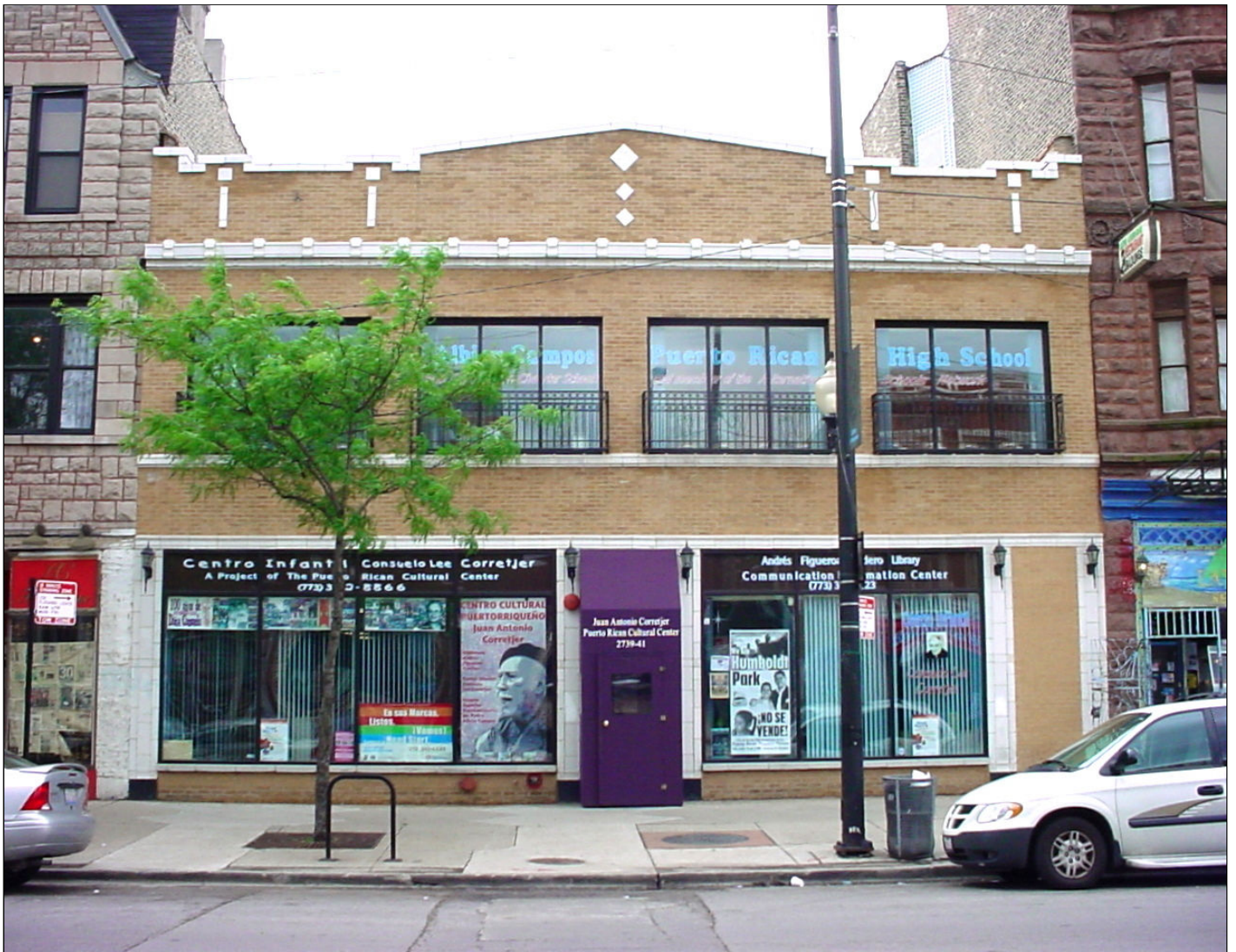
Humboldt Park neighborhood. Division 2739W, Chicago, Illinois.
