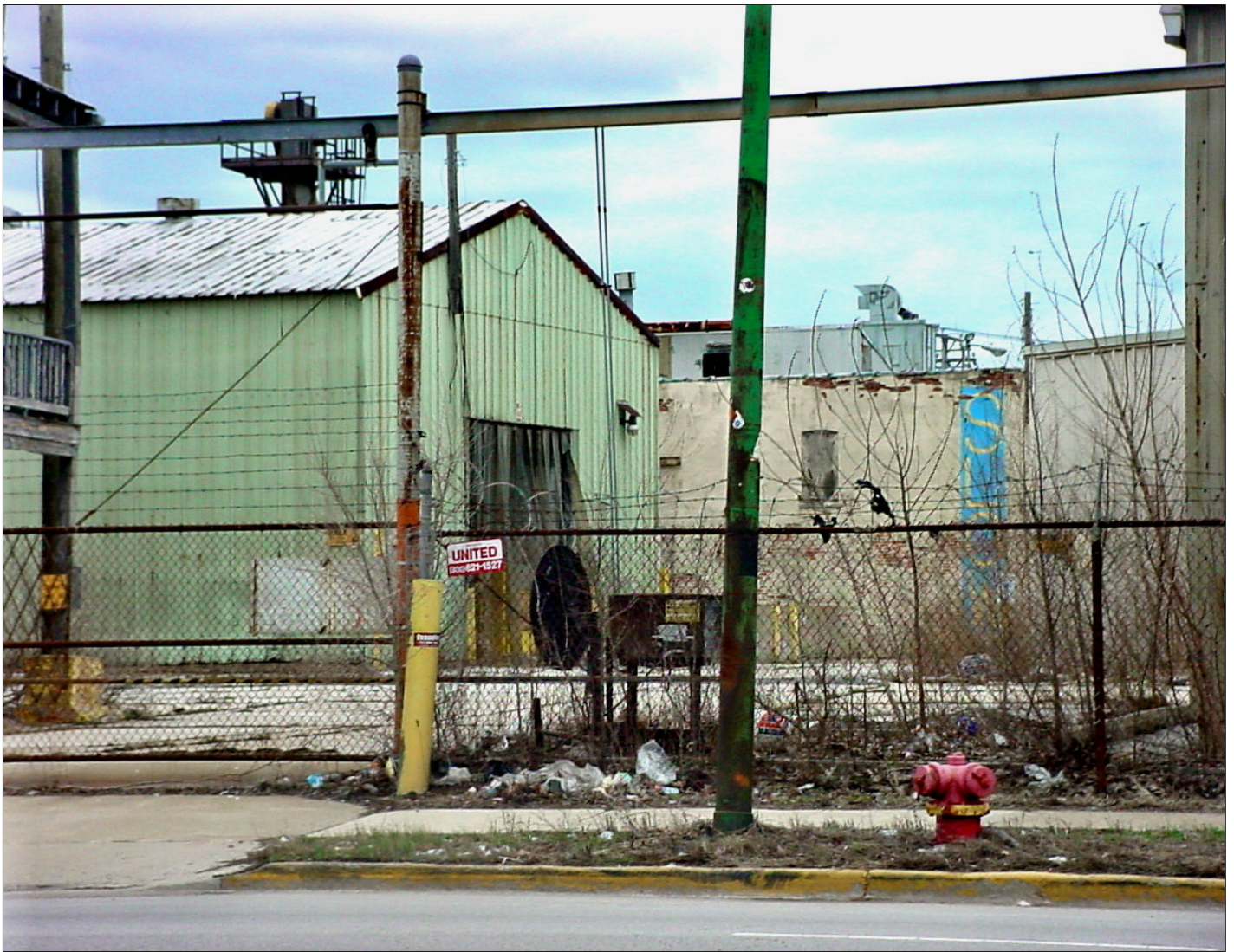
2008-04-11 Chicago Fire Brick Company. Ashland 7531S, Chicago, Illinois.
