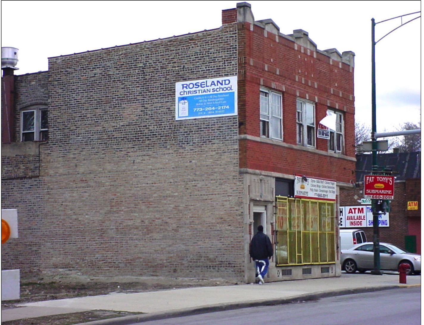
2008. Example of foreclosure and tax delinquent devastation, mid to far south side, Chicago, Illinois.
