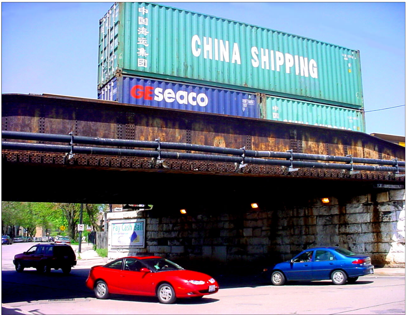
Underpass. Cermak 3400W, Chicago, Illinois.
