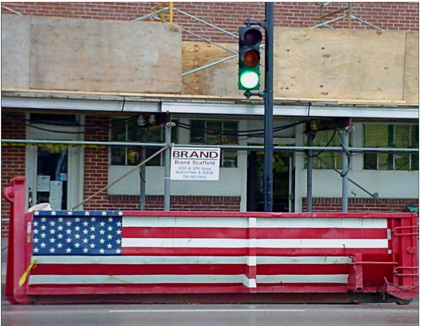
Small factory rehab financed by city loan. Cicero 2600N, Chicago, Illinois.
