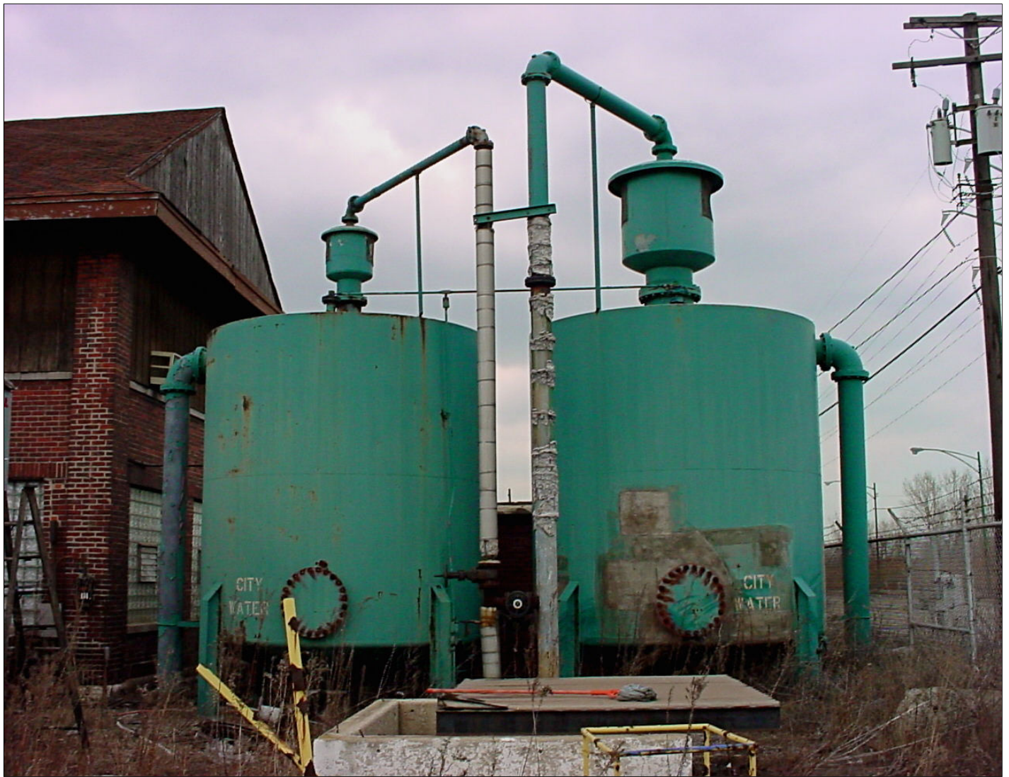
2005-02-23. Torrence Avenue 11236S. Acme Steel. Abandoned.
