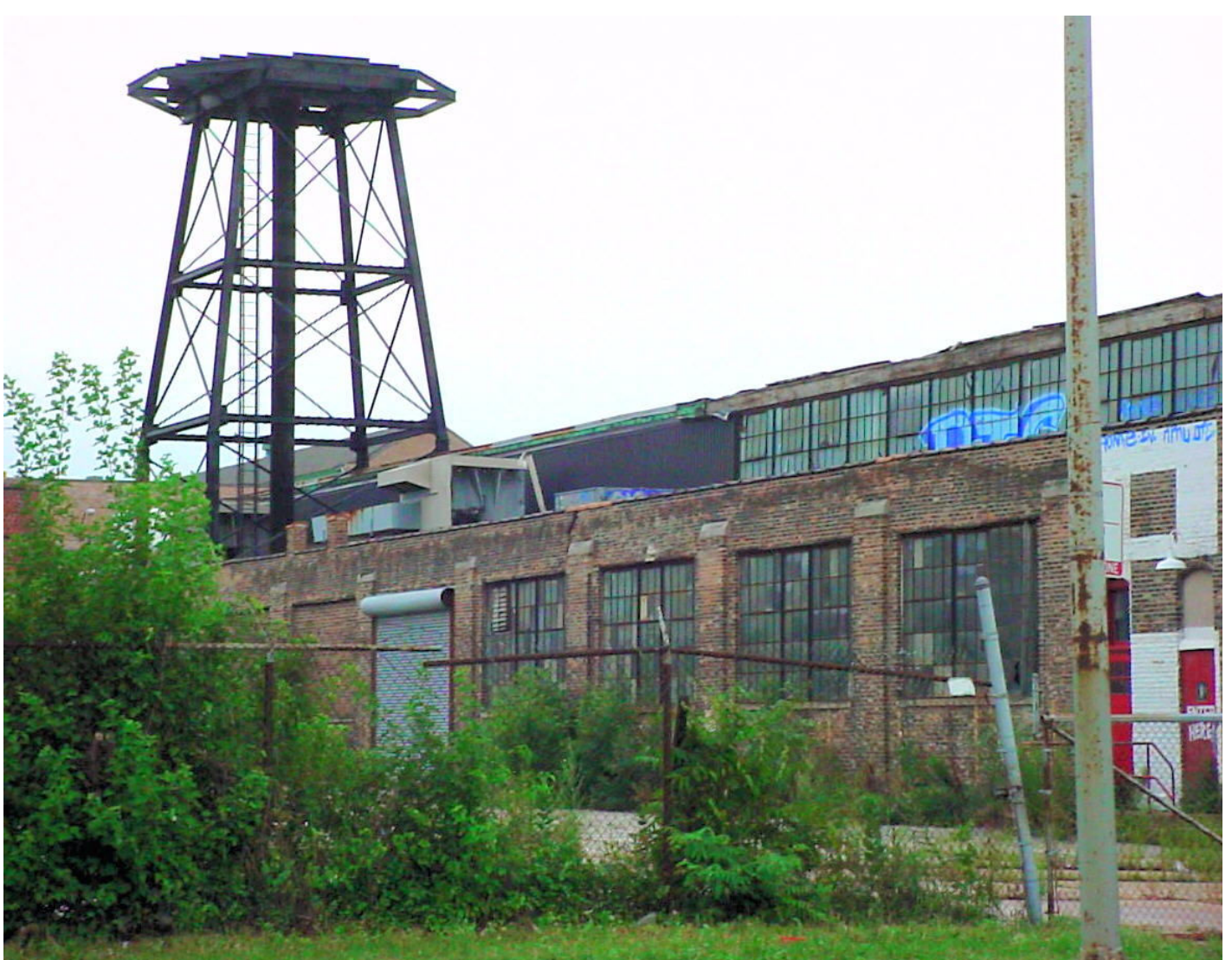
2004-08-25. Western Avenue 4500-4600S. Demolished.
