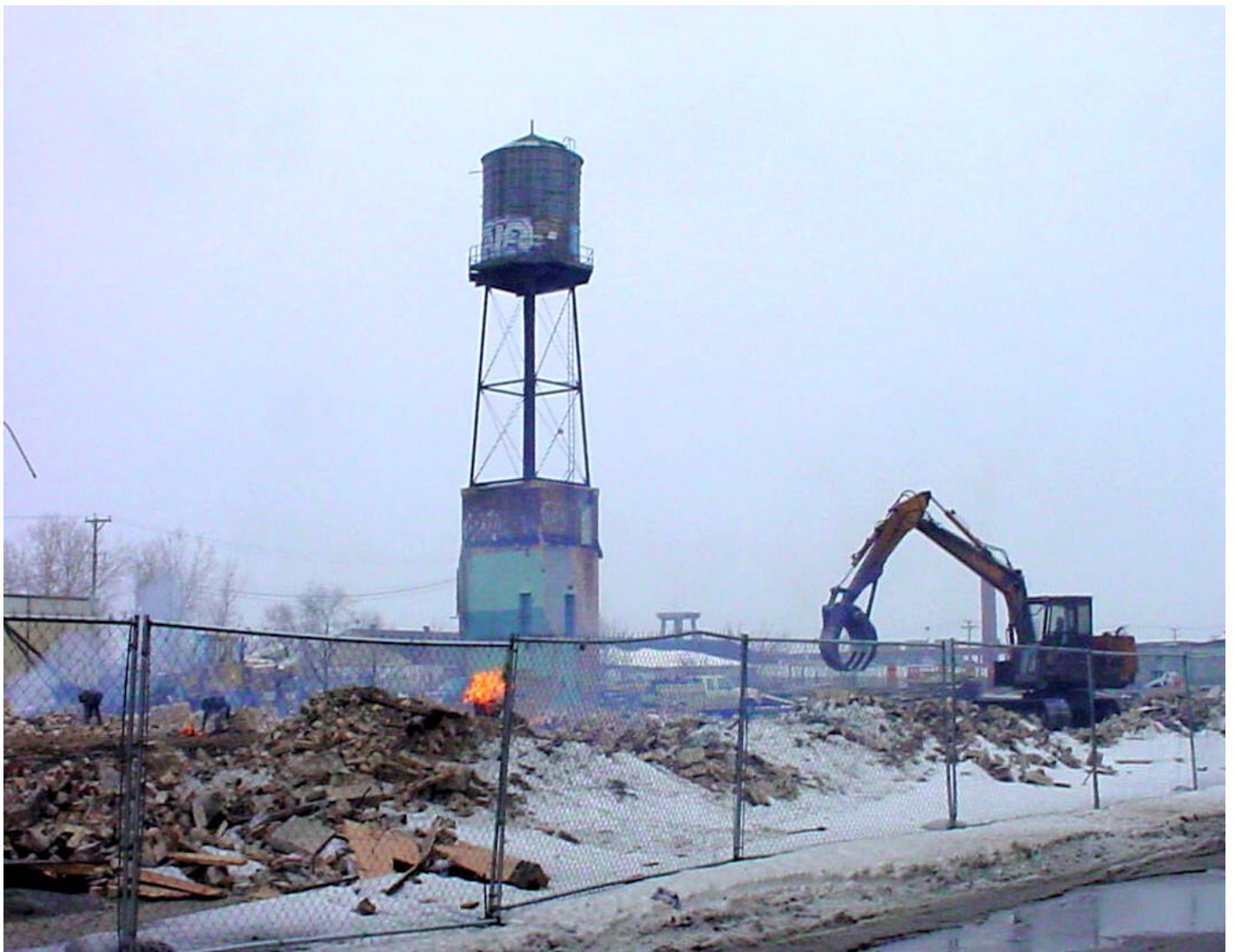
2005-01-26. Kedzie Avenue 4800S. Industrial conversion to (?). Rudd Container etc. Demolition days.
