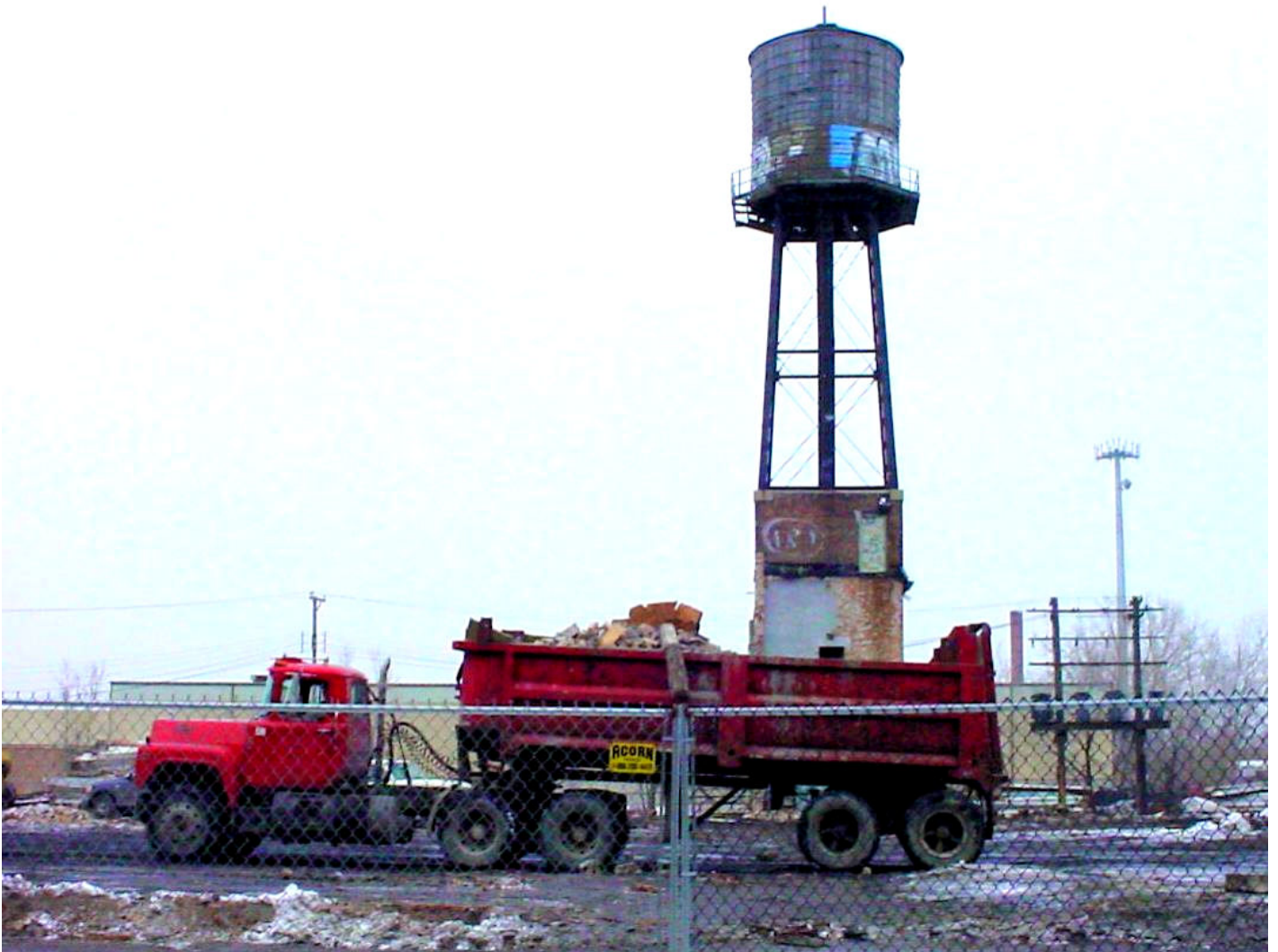
2005-01-26. Kedzie Avenue 4800S. Industrial conversion to (?). Rudd Container etc. Demolition days.
