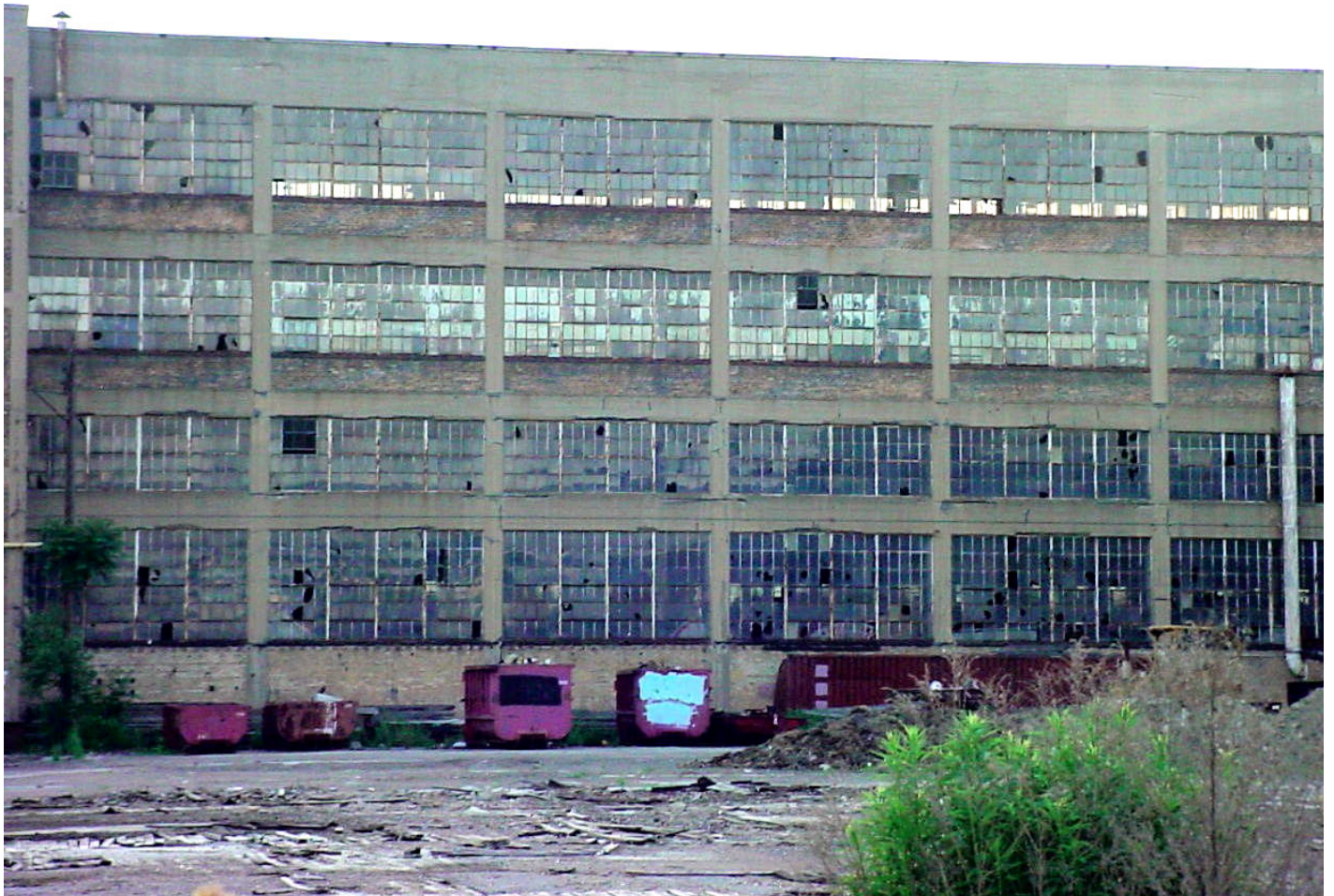
2005-06-10. Halsted St 4800S. Industrial park.. Abandoned.
