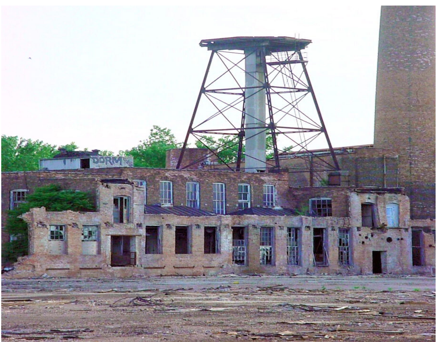
2005-06-10. Halsted S 4800S. Industrial park. Abandoned.
