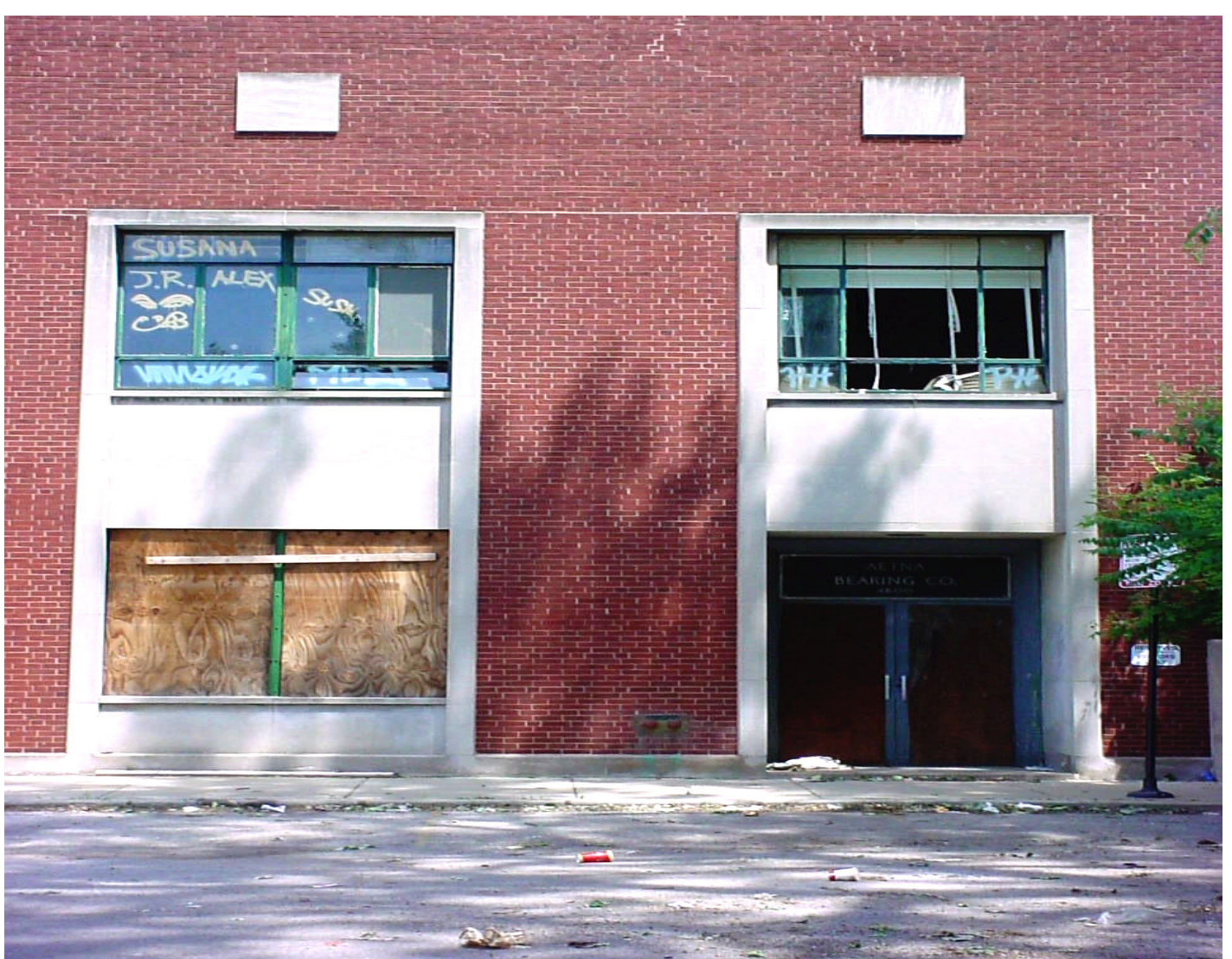
2005-06-07. Schubert 4600W. Aetna Bearing. Abandoned. Demolished 2007.
