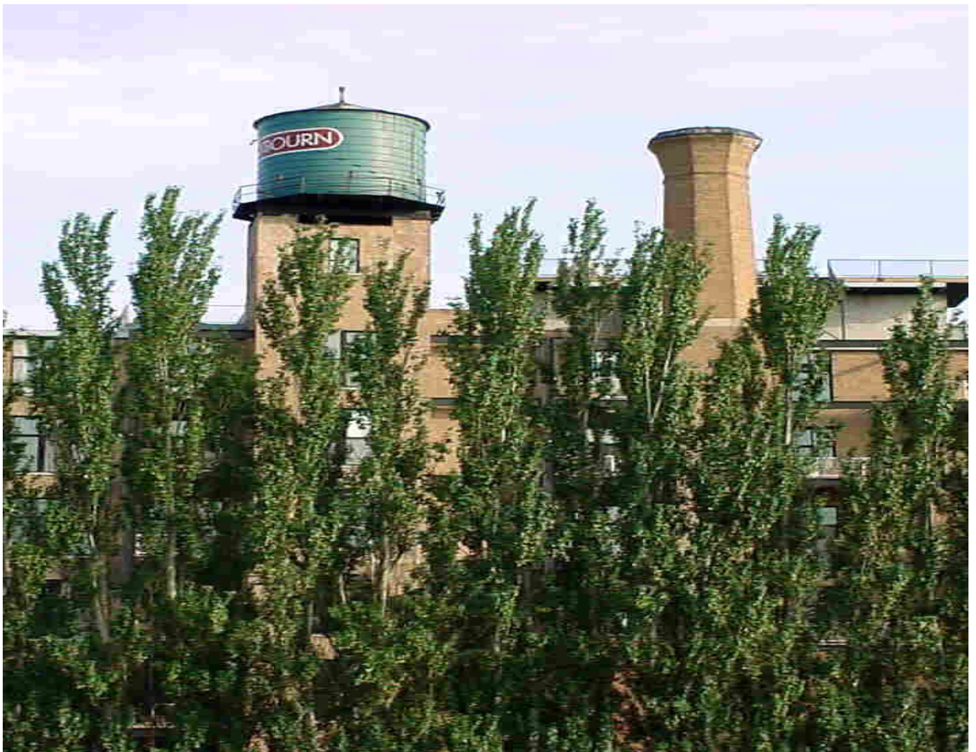
2003-03-23. Industrial/warehouse to residential conversion. Clybourn Avenue 1900N, Chicago, Illinois.
