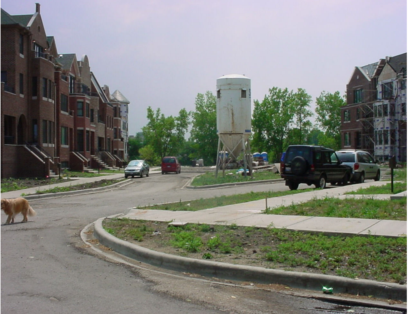
2005-06-29. Industrial park to townhome conversion. Racine Avenue 3300S, Chicago, Illinois. People are paying a lot of money to live in Dogpatch.
