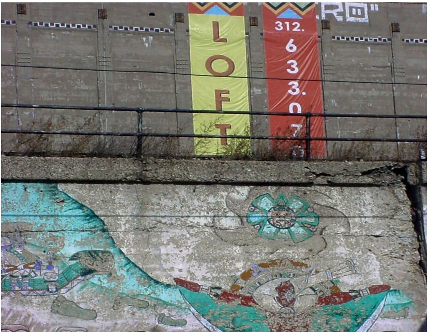
2005-03-06. Wholesale food market converted to residential. Loft buyers will get a property tax break. Blue Island 1360S, Chicago, Illinois.
