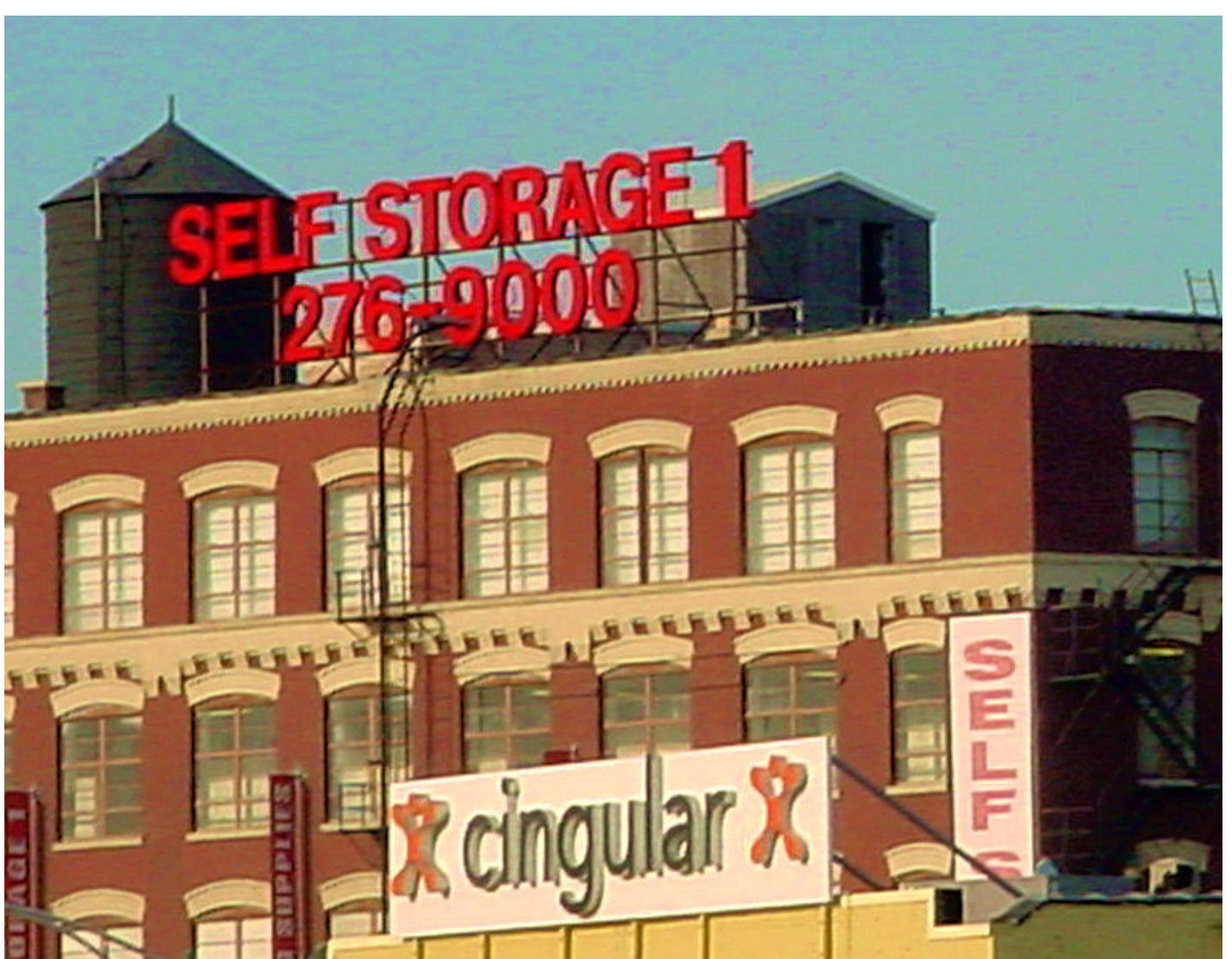
2005-02-12. Industrial building converted to storage. Elston Ave 2000N, Chicago, Illinois
