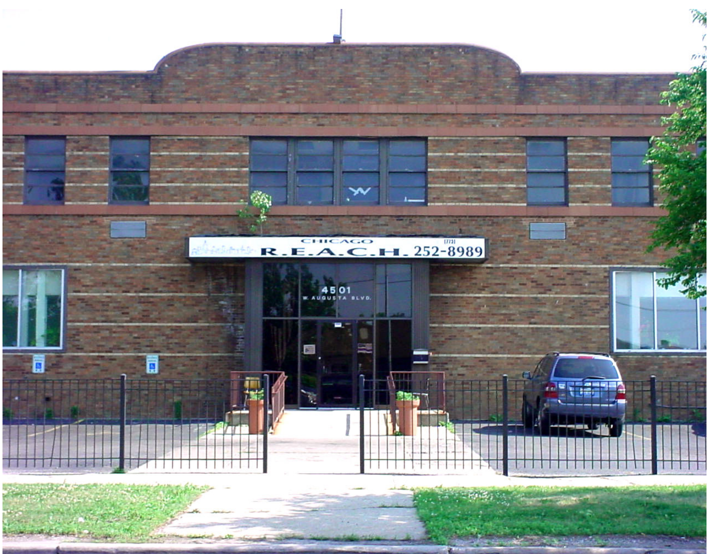
2005-06-10. Industrial to social service office conversion. Augusta Street 4501W, Chicago, Illinois.
