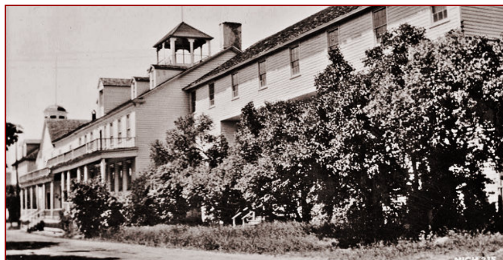
American Fur Company Buildings, Mackinac Island, MI. Norton, Charles, Jr. (photographer) (1936) HABS MI-215 https://cdn.loc.gov/service/pnp/habshaer/mi/mi0100/mi0120/photos/089347pv.jpg
