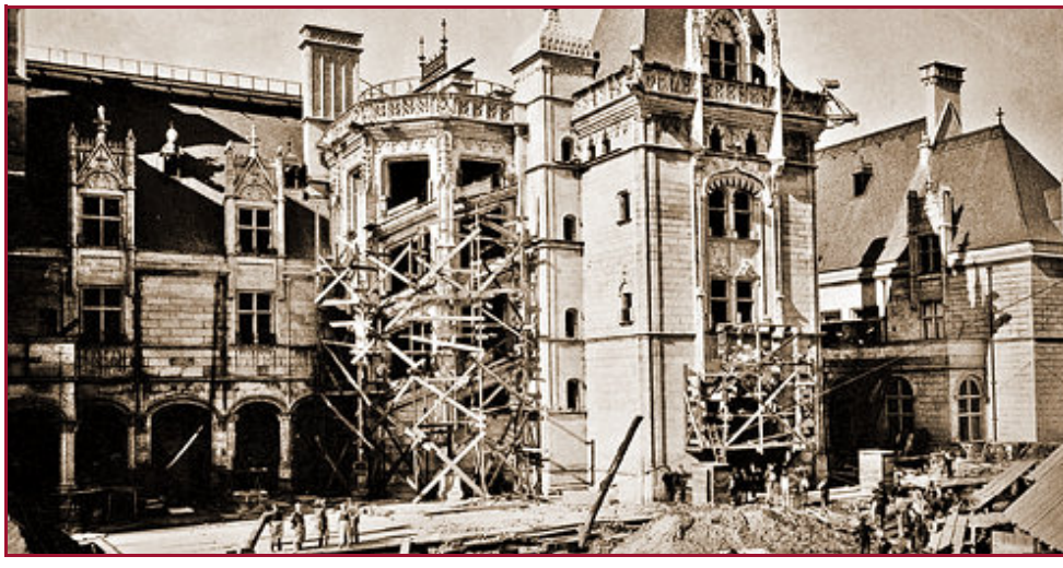
Biltmore castle under construction in Asheville, North Carolina (1889-1895) https://biltmore.s3.amazonaws.com/44510/con_bh_construction_facade-small_850x563__large.jpg
