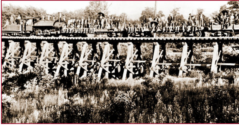
Private railroad for construction of Biltmore castle https://biltmoreestatebyzli.weebly.com/uploads/2/4/6/0/24601956/1746288_orig.jpg
