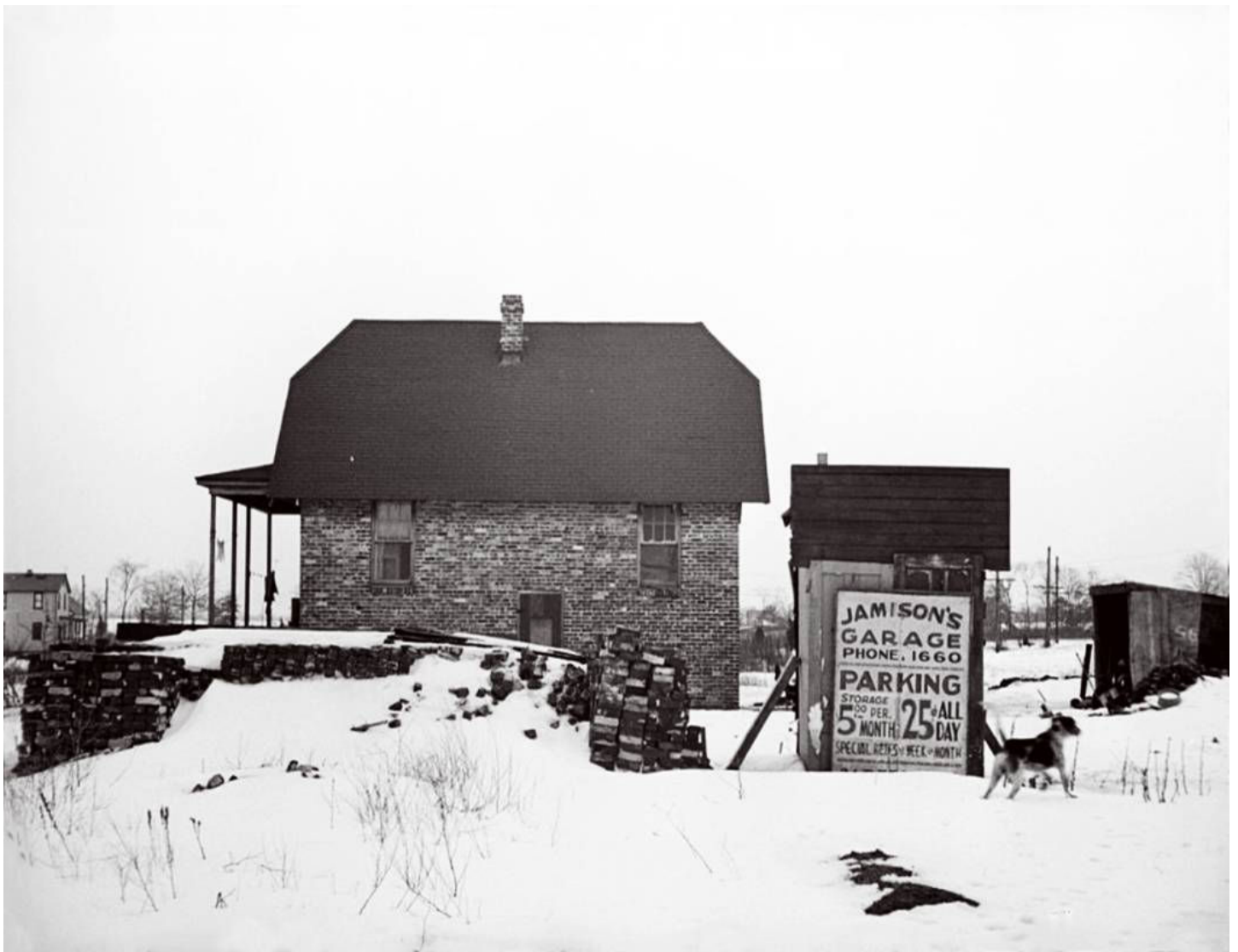
Mydans, Carl (photographer). House off Lincoln Highway, Franklin Township (Somerset County), Bound Brook, New Jersey. 1936 February.
