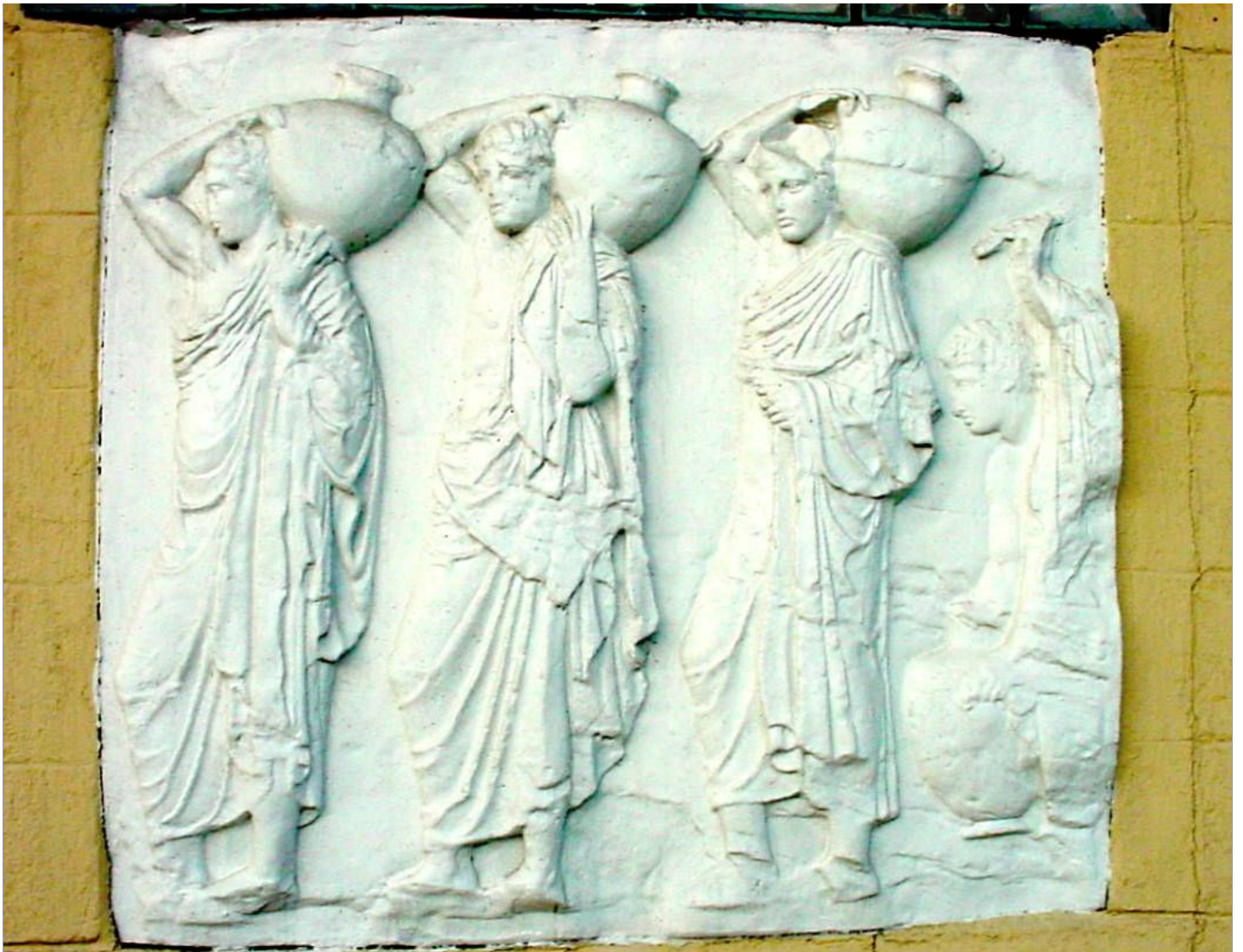
Restaurant (south wall). Hubbard at Union (northwest corner). Chicago, Illinois.
