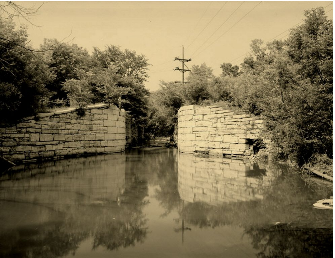
Gooding, William. I&M Canal Lock #2, located about one mile south of Lock #1, in Lockport. Historic American Engineering Record. HAER ILL,99-LOCK,2-9. Lockport Historic District, Illinois & Michigan Canal, Lockport, Will County, IL
