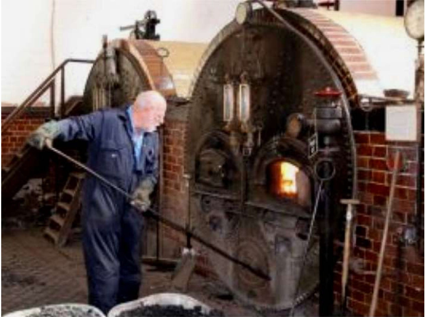
Boiler Room. Papplewick Pumping Station, Nottinghamshire, England.
