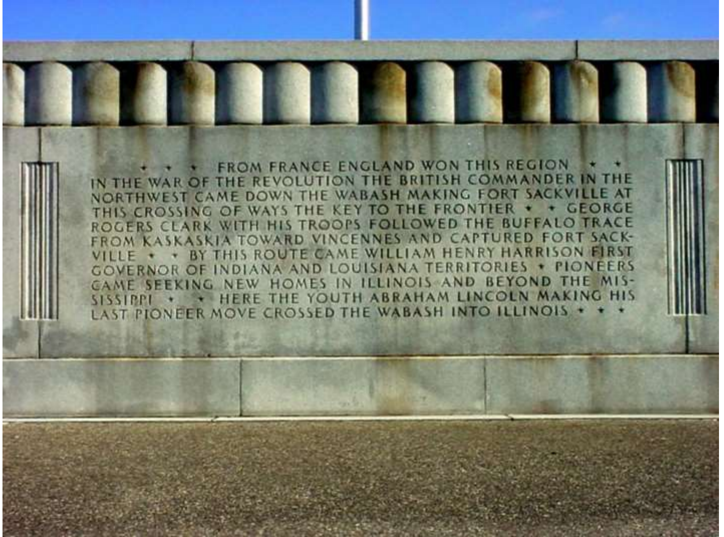
Jefferson Memorial Bridge. Vincennes, Indiana. (2008 January 15)
