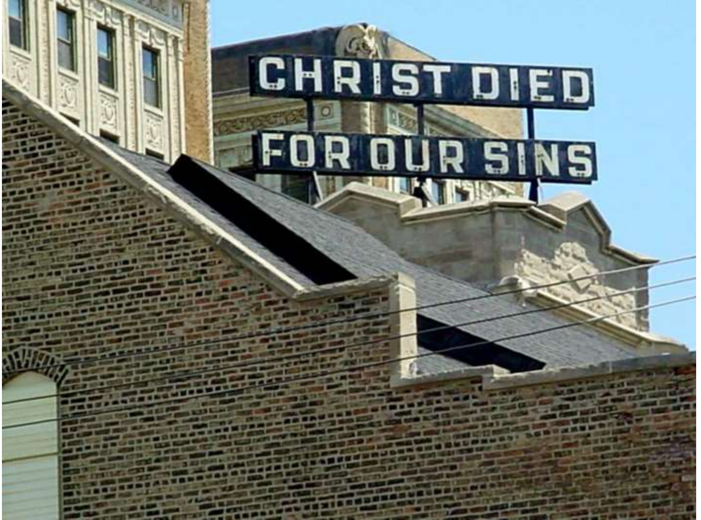
Stewart Elementary School Sunnyside at Broadway (behind sign on church at Wilson & Sheridan). Chicago, Illinois (2010 June 29).
