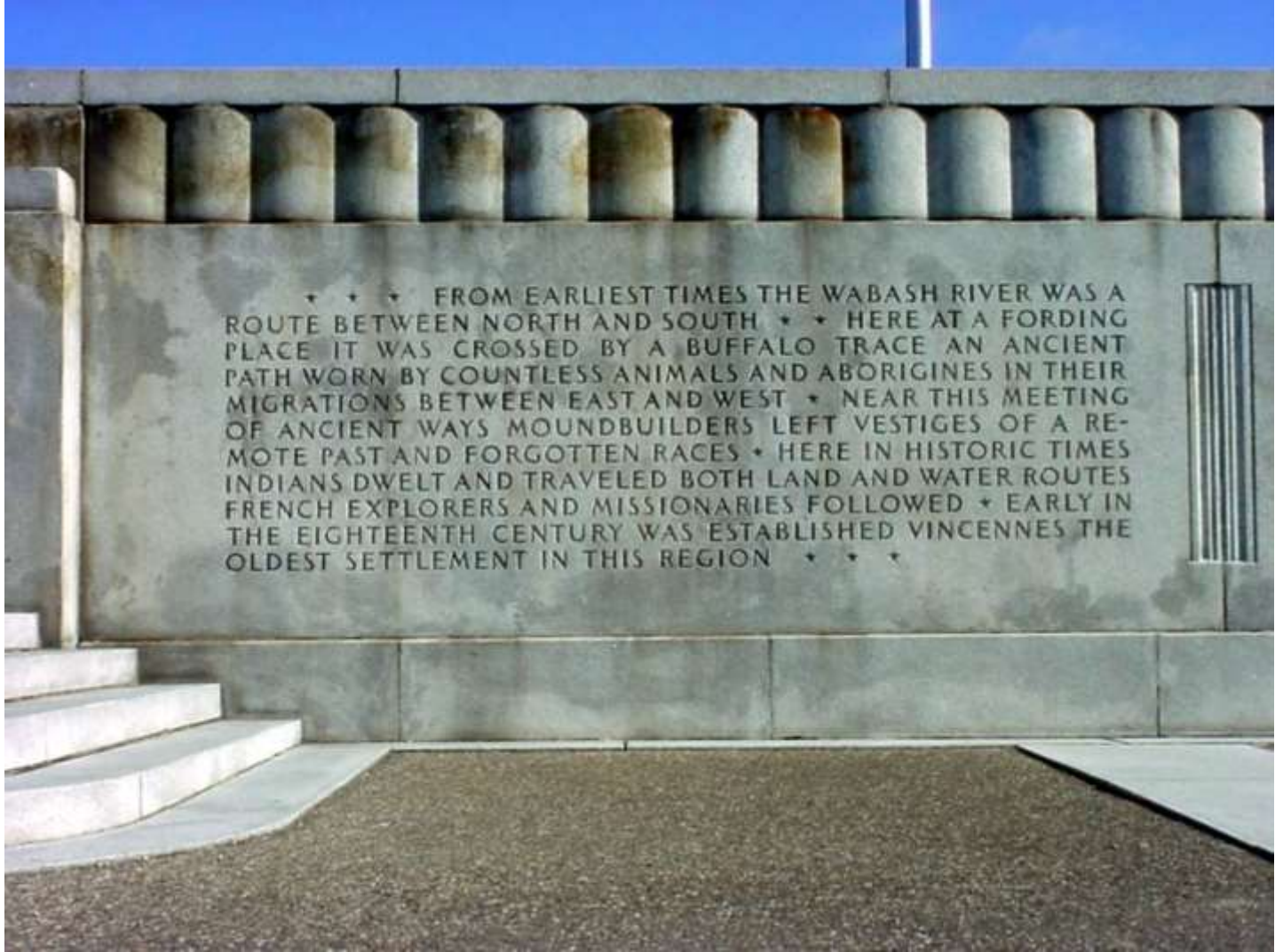
Jefferson Memorial Bridge. Vincennes, Indiana. (2008 January 15)
