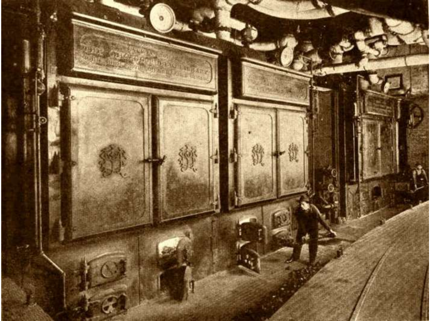
Furnace room and man with shovel. Chicago Public Library, Chicago, Illinois (1902).
