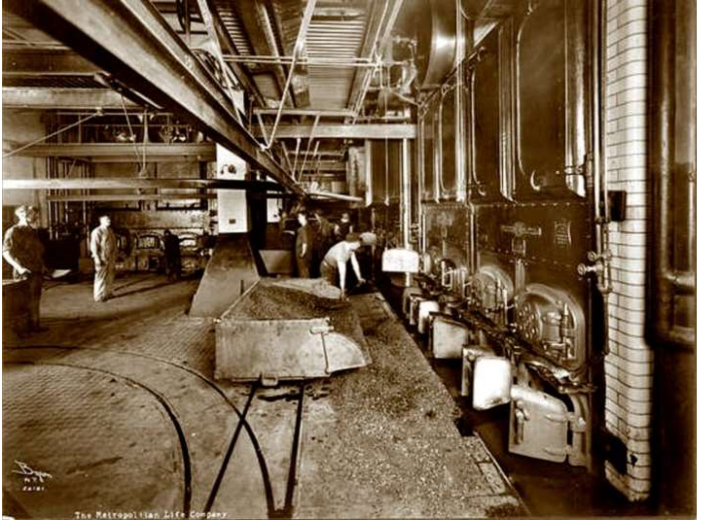
Men shoveling coal into the furnaces/boilers. Metropolitan Life Insurance Co. 23rd at Madison. New York, NY (1907).
